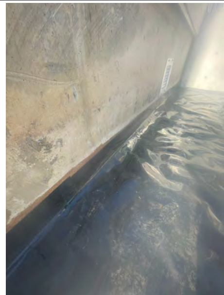
An overview of the retrofit detailing.
