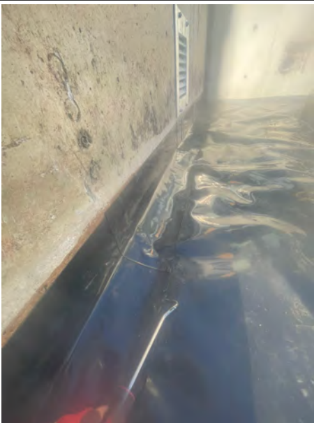
A pick and probe test being conducted upon retrofit detailing.
