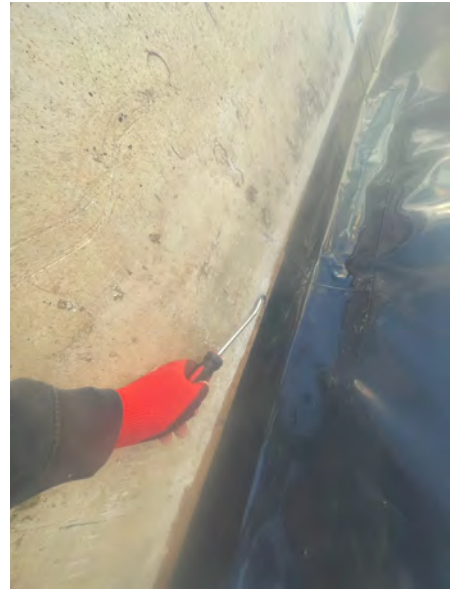
A pick and probe test being conducted upon the retrofit detailing.
