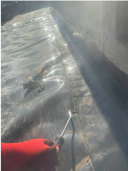
A pick and probe test being conducted upon a welded lap joint.
