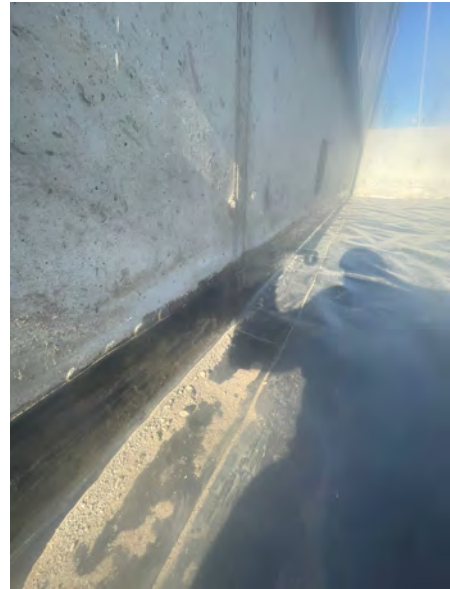
An overview of the retrofit detailing.
