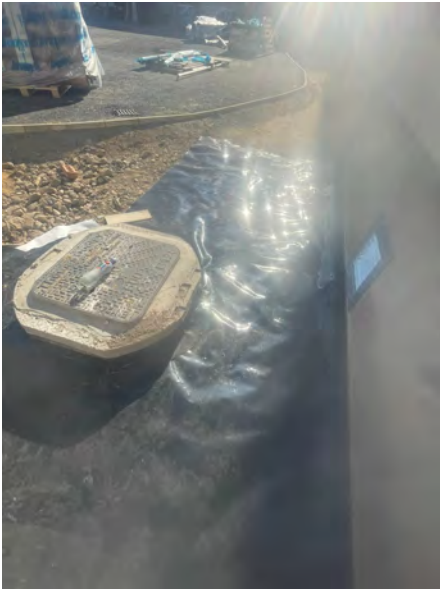
A sealed manhole.
