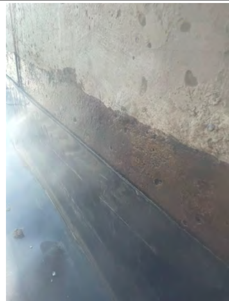
An overview of the retrofit detailing.
