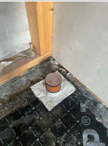
A sealed pipe penetration.
