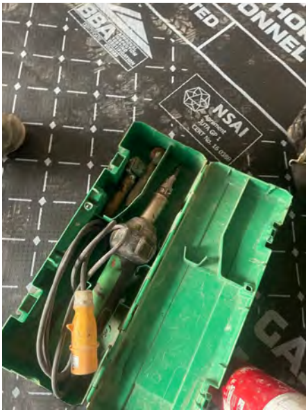
A hot air leister and silicone roller used on site.
