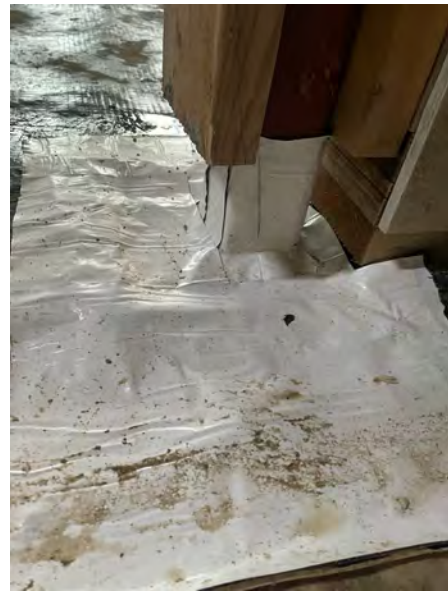
A sealed corner detail.
