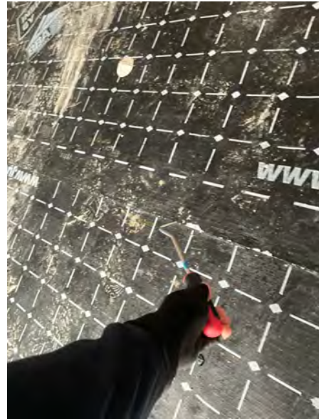
A pick and probe testing being carried out.
