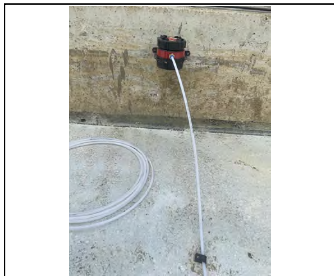
Ground gas monitor fixed.
