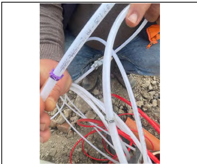
Probe pipe individually tagged.
