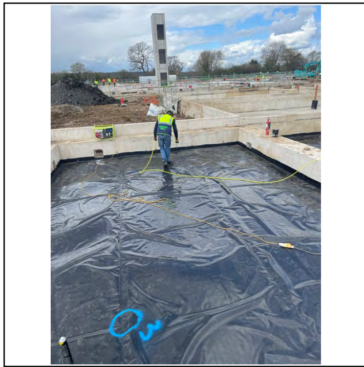
Airlance integrity testing to welded lap joint.
