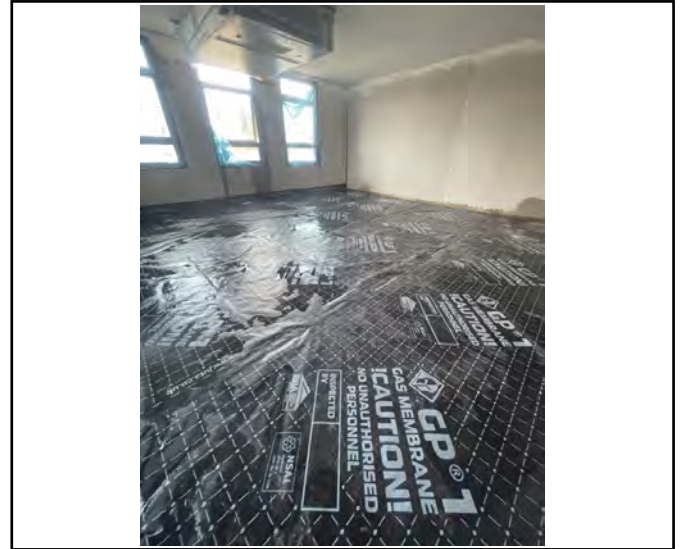
Internal overview photograph.
