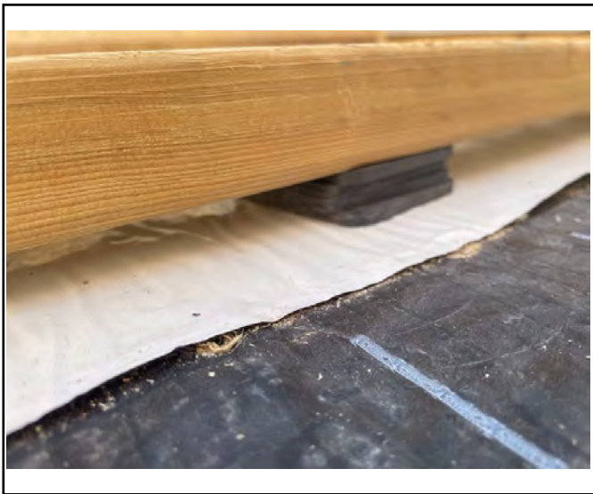
Evidence of GPSAM beneath
