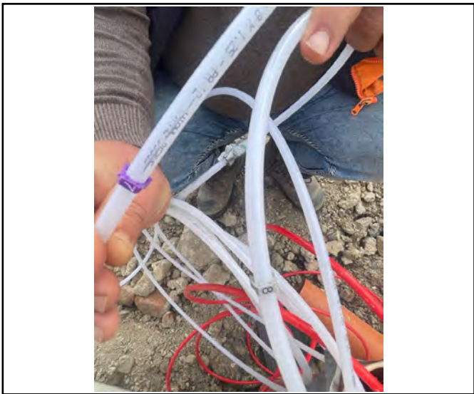
Probe pipe individually tagged.
