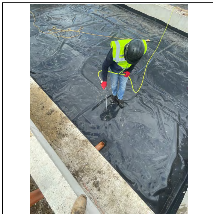
Airlance integrity testing to sealed pipe.
