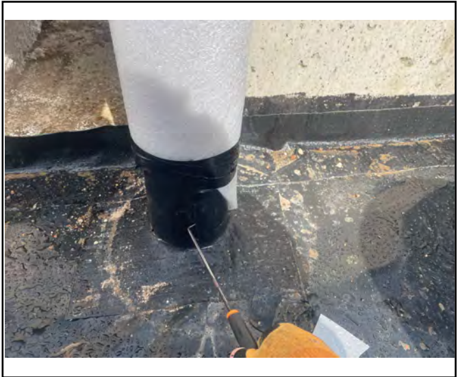
Pick&probe testing to sealed pipe.
