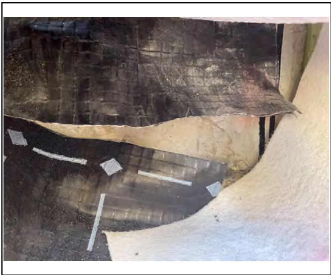
Unsealed and inadequate overlap.
