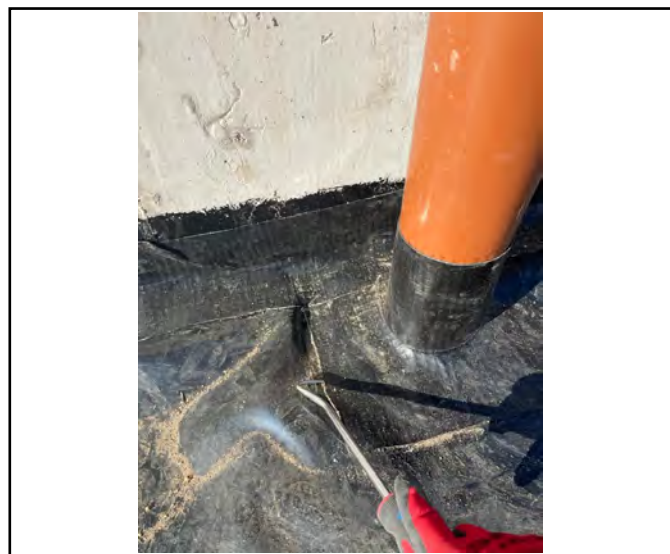
Pick&probe testing to sealed pipe.
