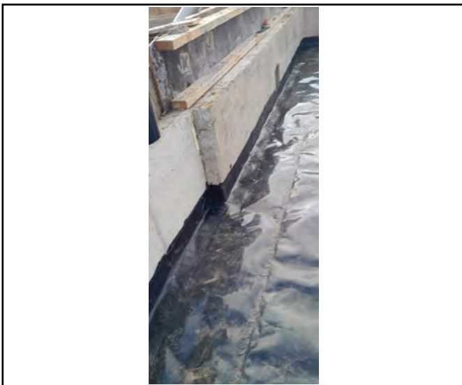
Installation of the retrofit dealing required onsite.
