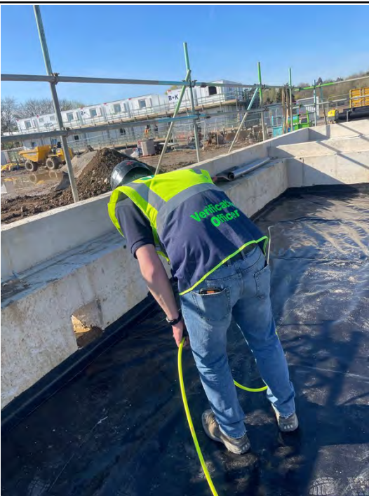
Airlance integrity testing to welded lap joint.
