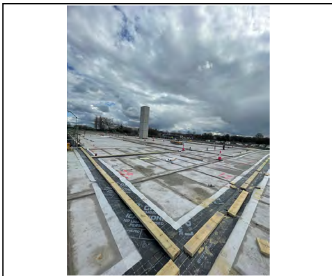
Juta GP1 perimeter and internal wall
