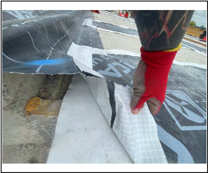
Dual taped lap joint evidence.
