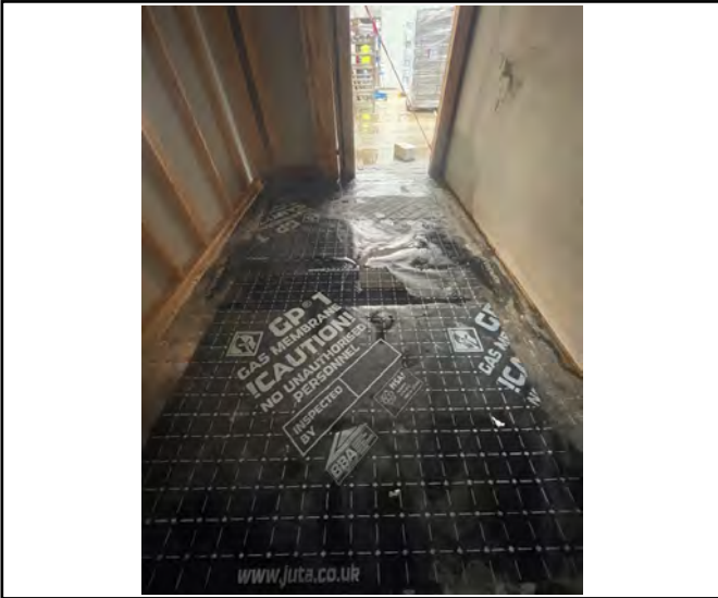
Internal overview photograph.
