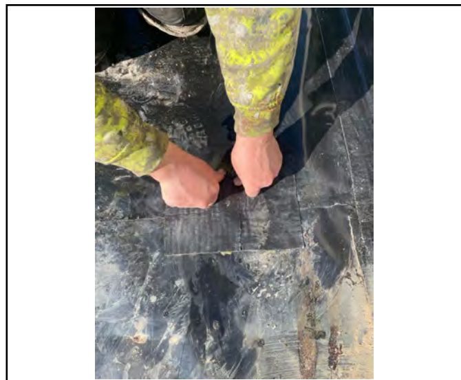
Installer carrying out patch repair
