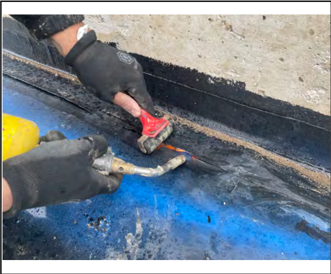
Heat applied to remediated area.
