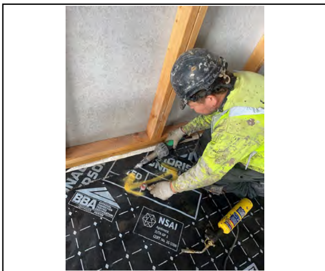
Re-welded remediation.
