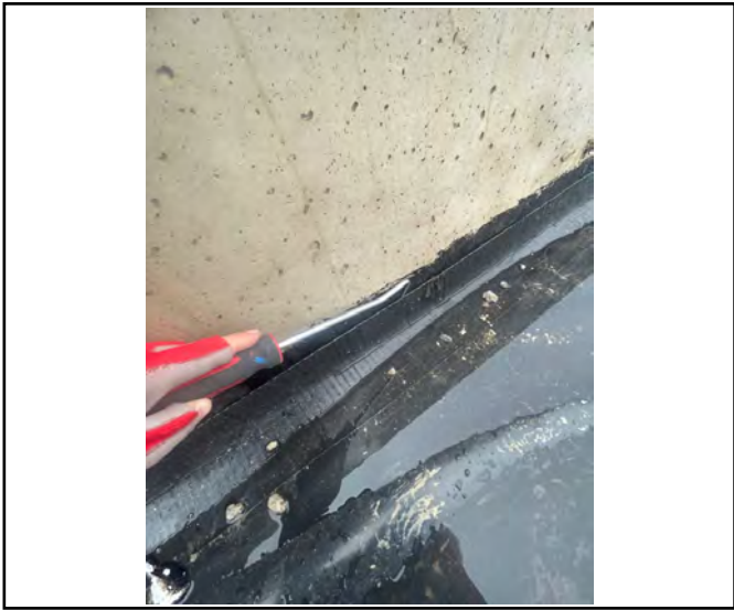
Pick&probe testing to retrofit detailing.
