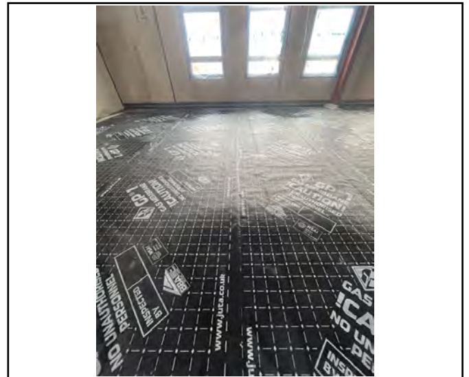
Internal overview photograph.
