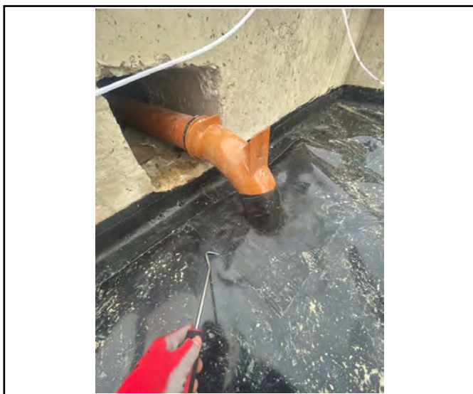
Pick&probe testing to pipe penetration.
