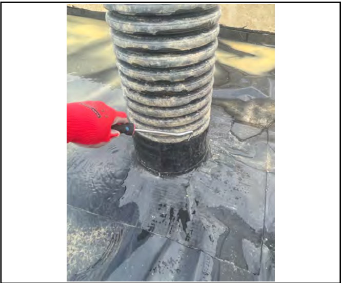
Pick&probe testing to pipe penetration.
