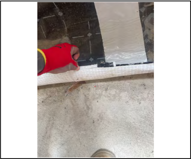
Dual taped lap joint evidence.
