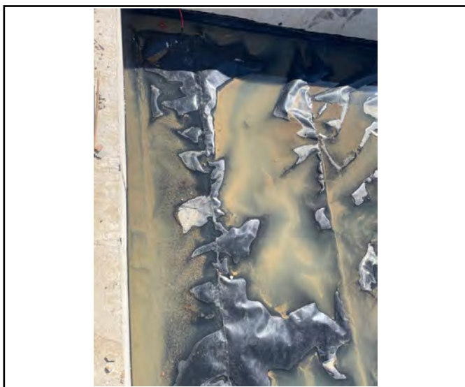
Cut membrane remediated from previous visit.
