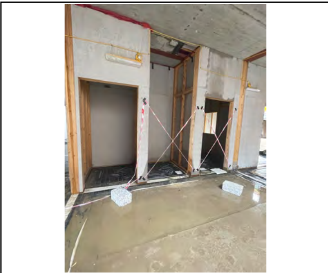
Internal overview photograph.
