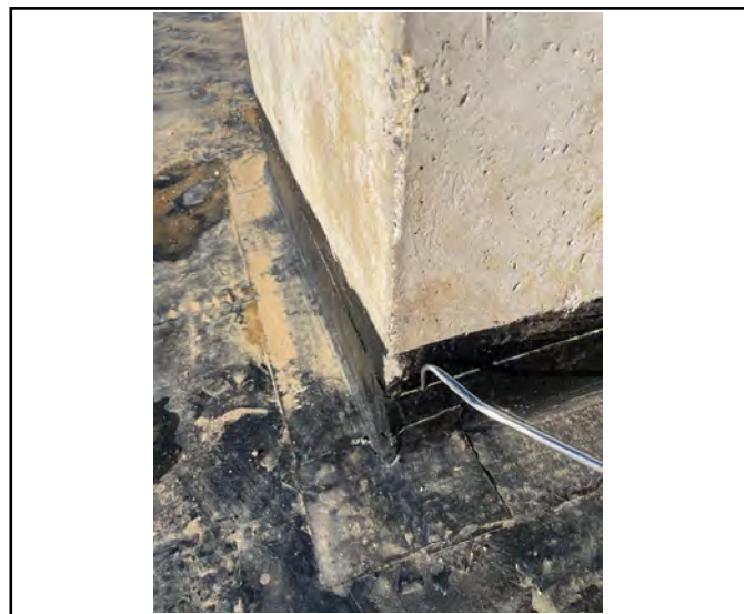
Pick&probe testing to retrofit detailing.
