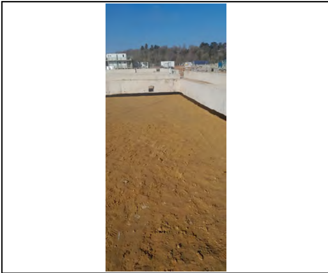
Photograph of the sand blinded floor ready for the membrane.
