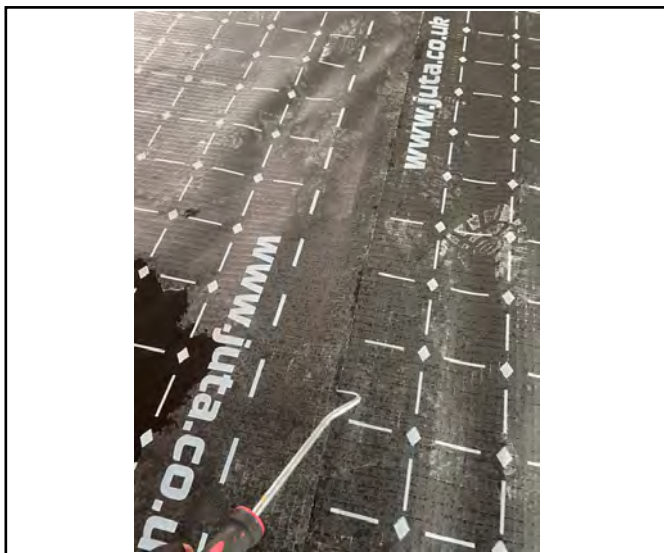
Pick&probe testing to welded lap joint.
