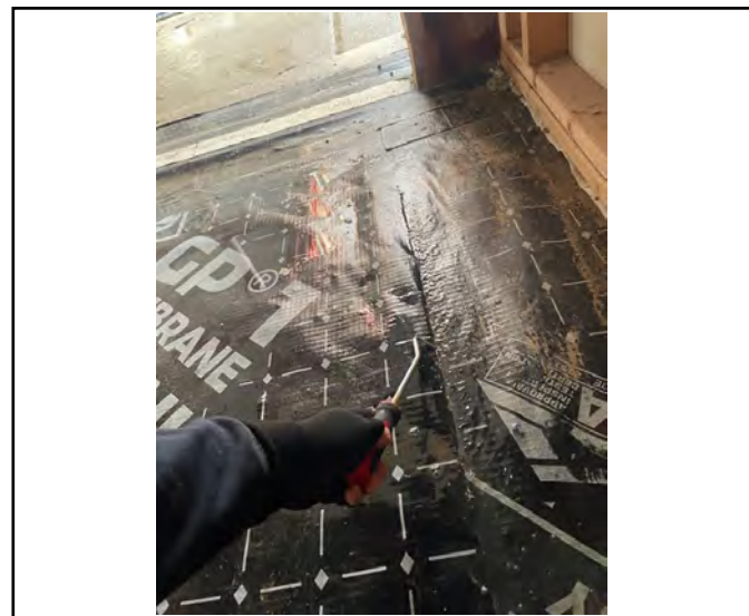
Pick&probe testing to welded lap joint.
