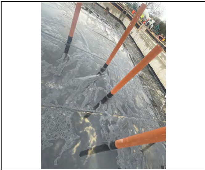
Successfully sealed pipe penetrations.
