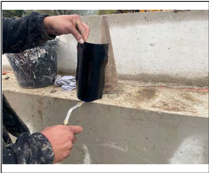
Heat applied to patch repair.
