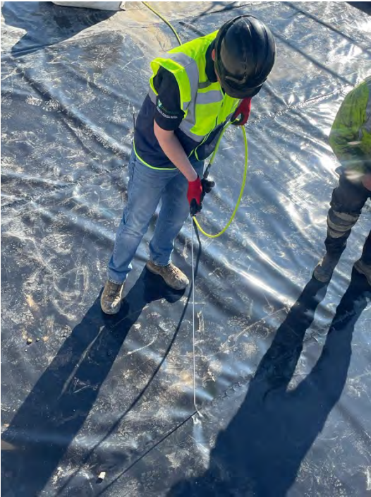
Airlance integrity testing to welded lap joint.
