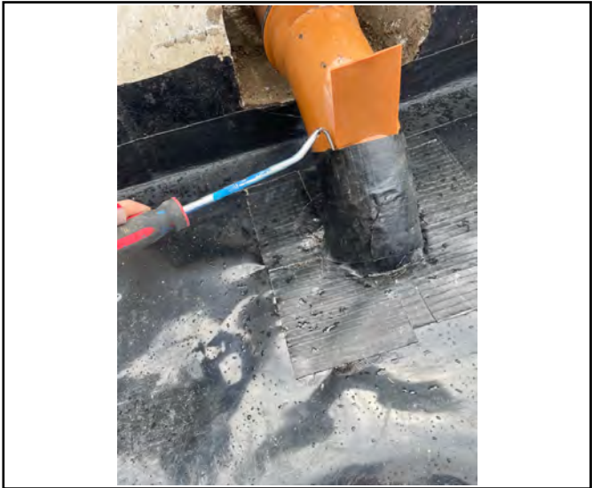
Pick&probe testing to sealed pipe.
