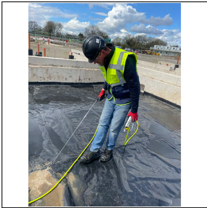
Airlance integrity testing to welded lap joint.
