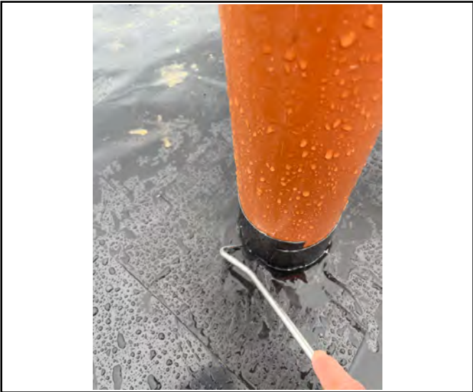
Pick and probe test carried out on a pipe penetration.
