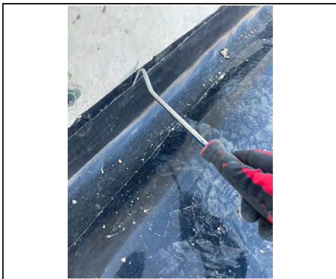
Pick&probe testing to retrofit detailing.
