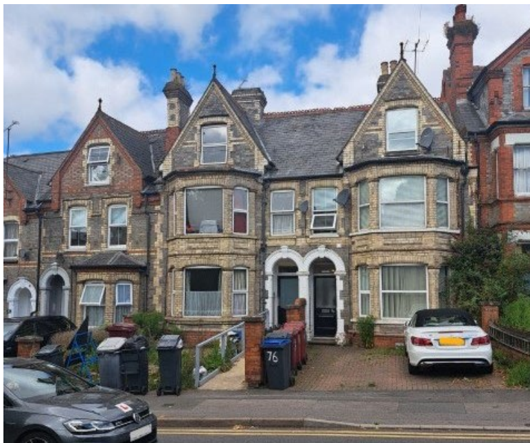
Photo 1 – View of the front elevation
