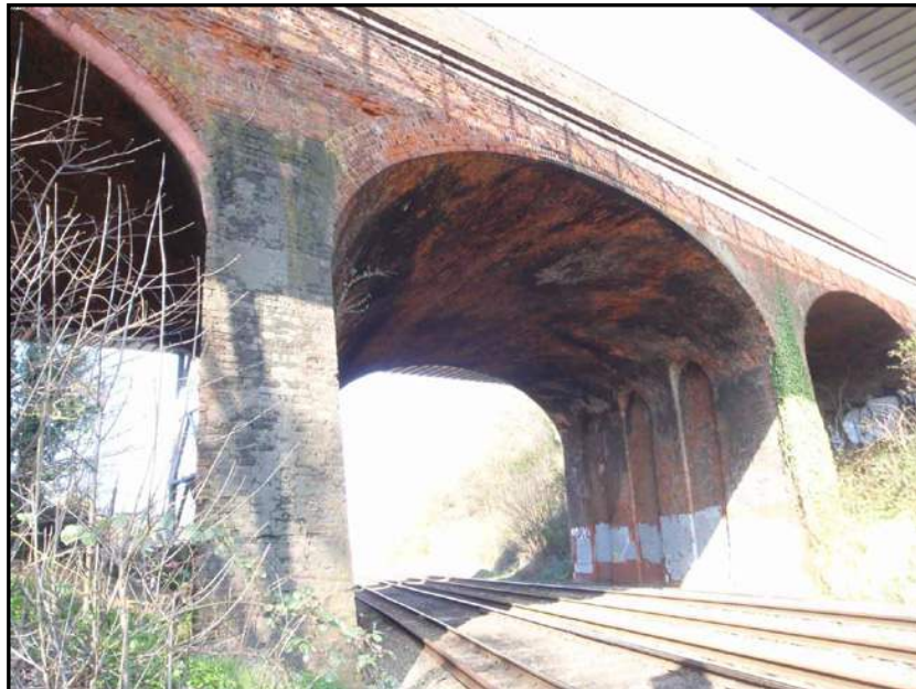
Figure 1: Bath Road Overbridge
