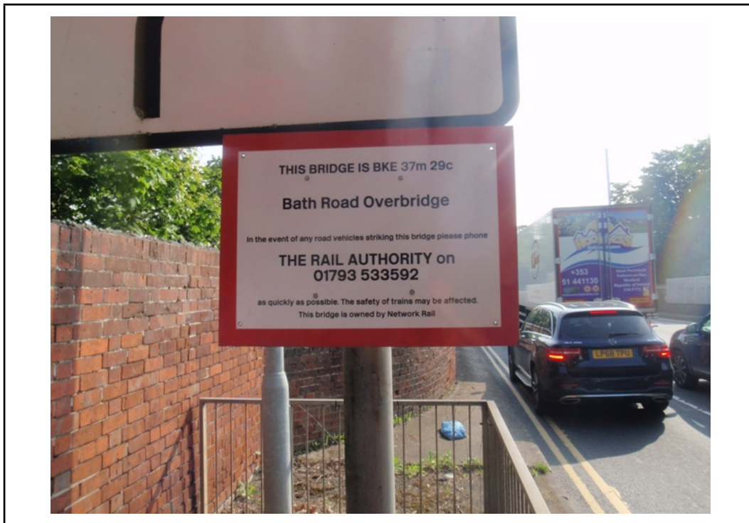
Photo No 3 - Bridge ID sign 11/05/24 -
