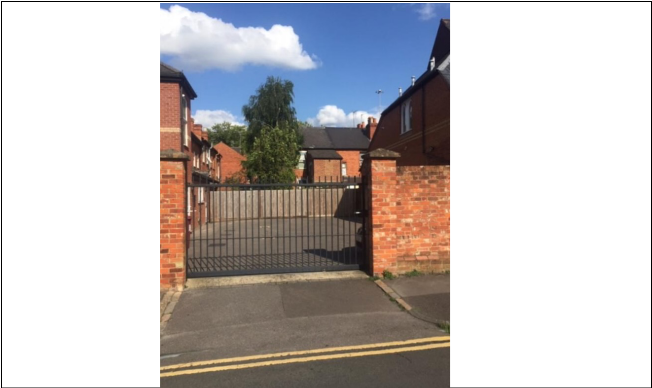
Rear elevation today to the right of the tree from Carey Street (rear of The Oasis)
