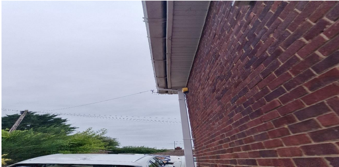
Picture 3: Showing the tight eaves
