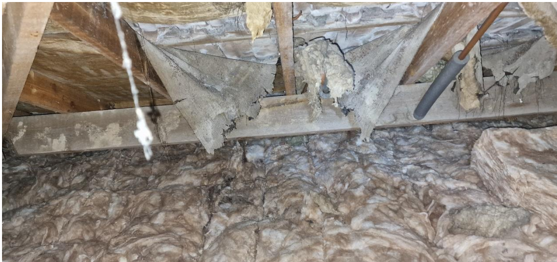
Picture 4: Showing the internal roof structure and the bitumen paper felt.
