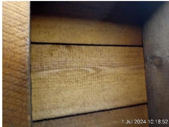
Figure 22: Example of tight timber lining in loft voids.
