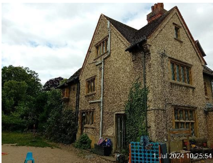
Figure 4: Rear of B1.
