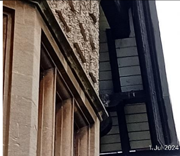
Figure 23: Example of tight timber eaves.
