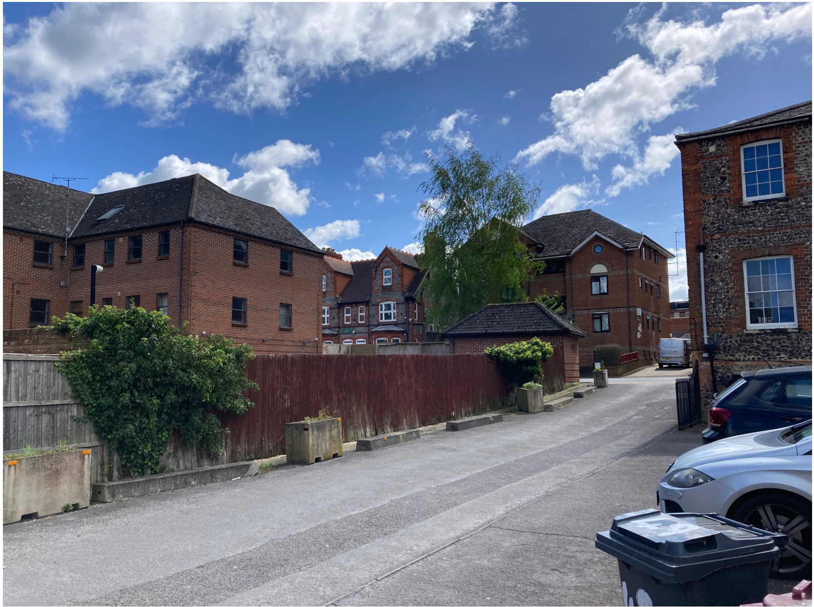
No 43 – 49 Livery Close from the rear and the existing building on the site
