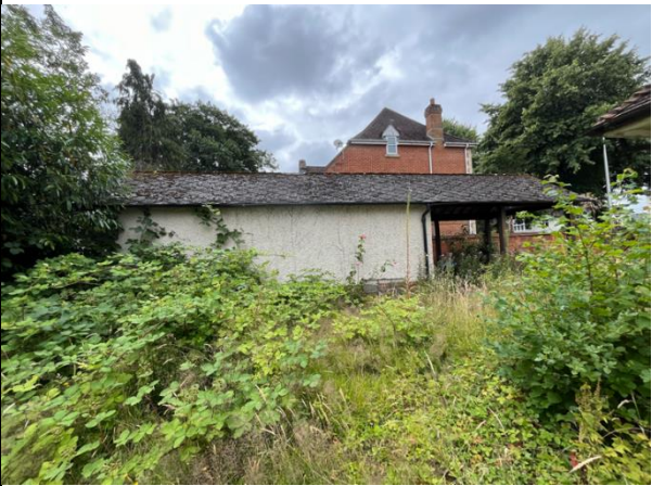
Photo 8 – southern elevation of building 2
