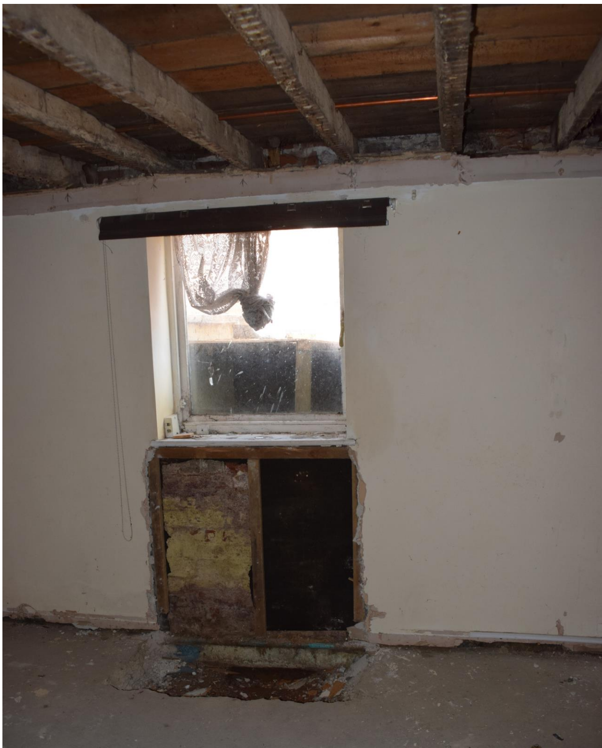
Plate 4 excavated area to the front of the building , seen internally
