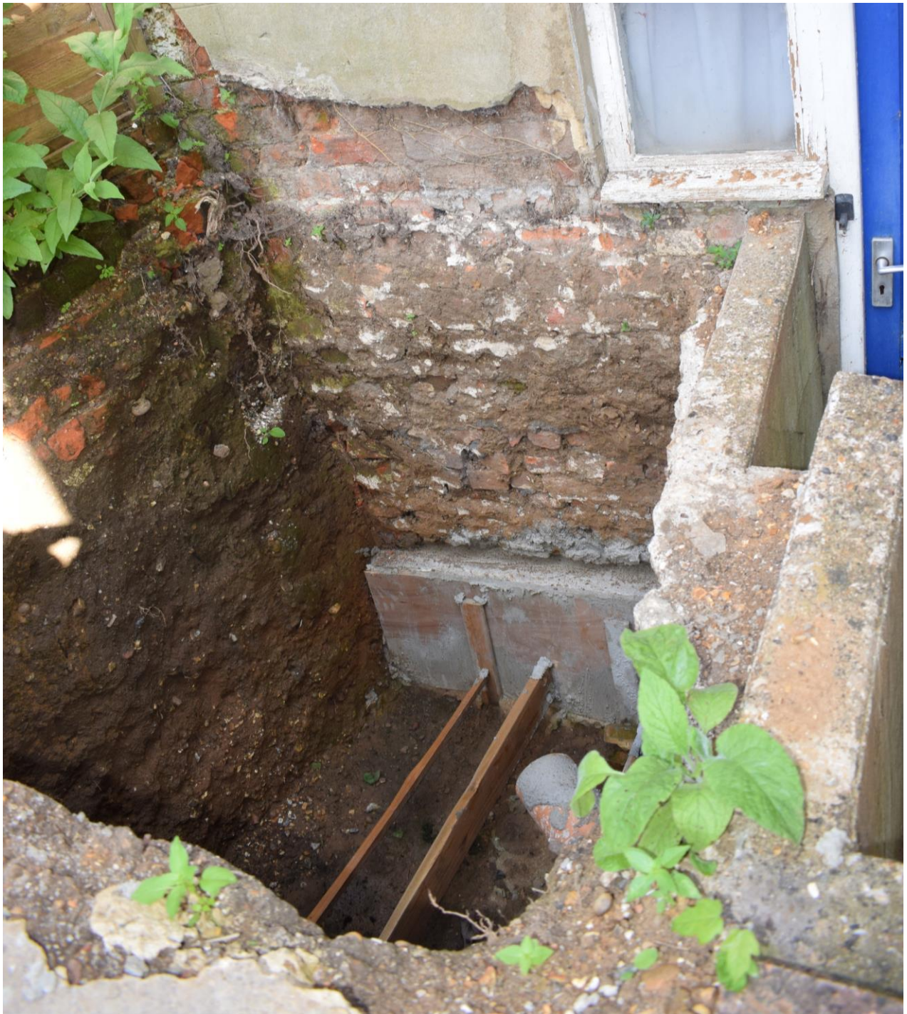
Plate 3 excavated area to the rear of the building
