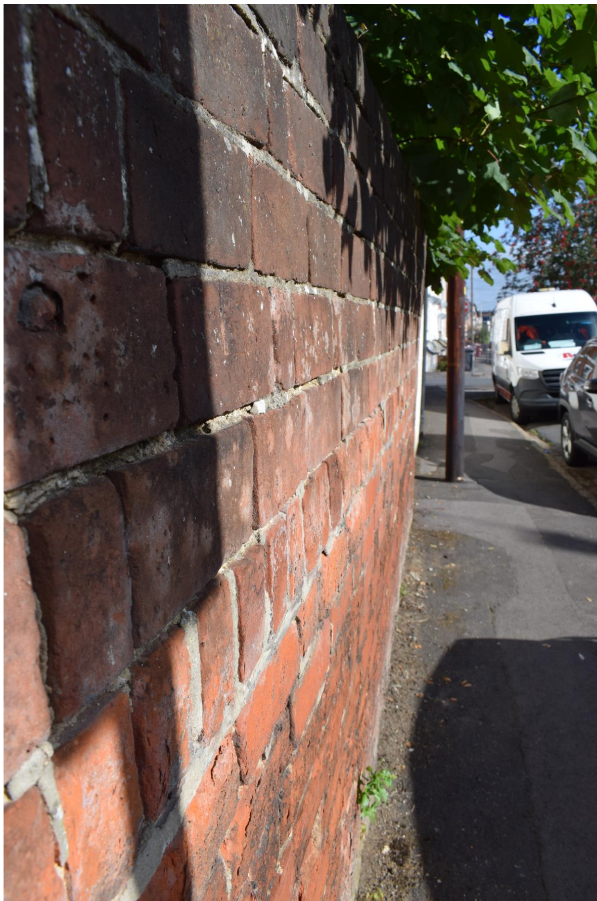
Plate 7 the increasing distortion of the garden wall
