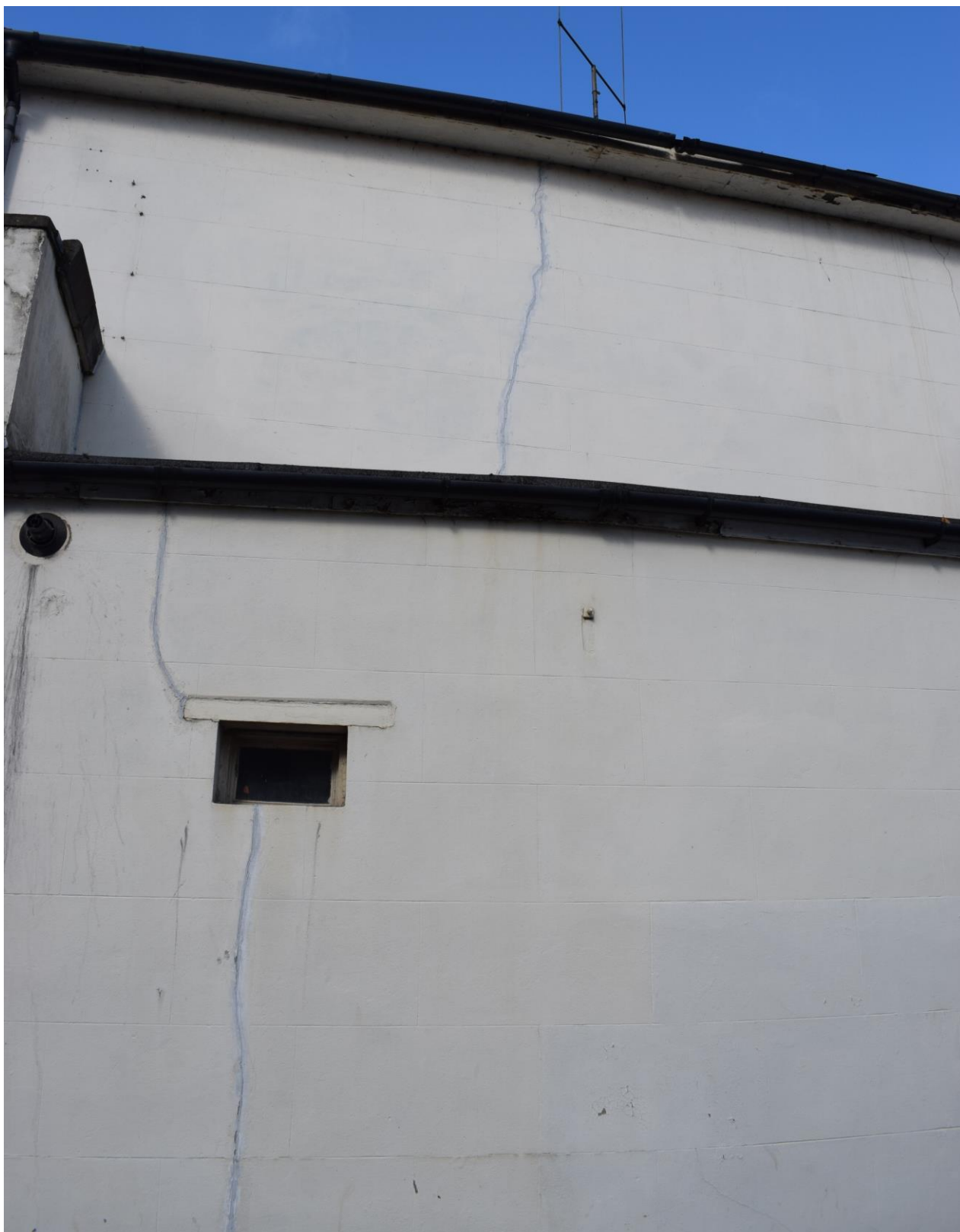
Plate 2 fractures in the render
