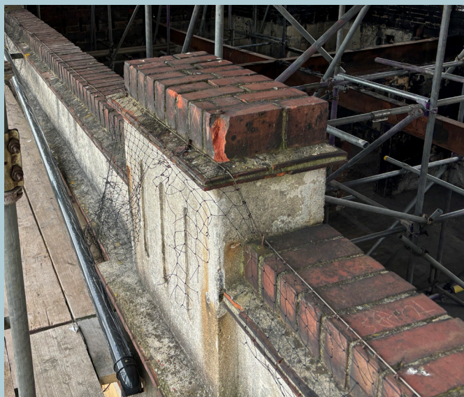
Figure 4: Brickwork Parapet Wall (© THP)
