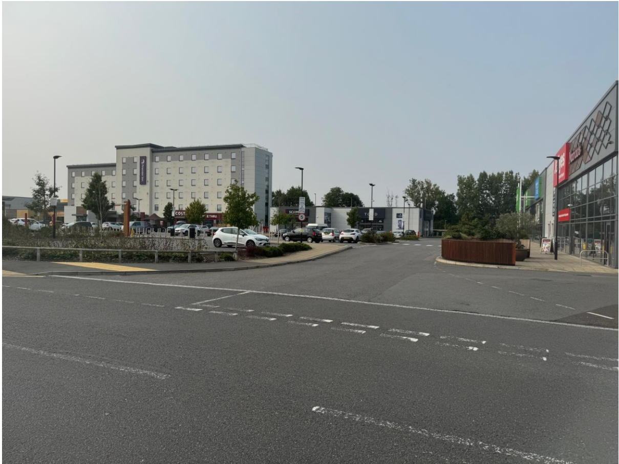
Site Visit Photos taken on 19 th of August 2024
