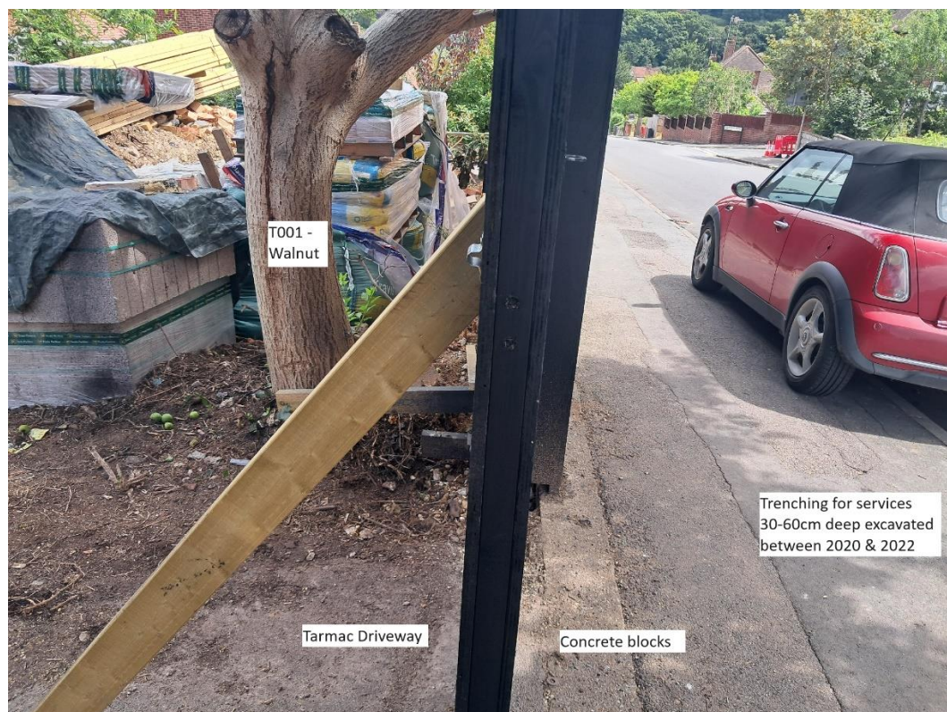
Images 8 – Existing development / trenching within the rooting area of T001 (Walnut)
