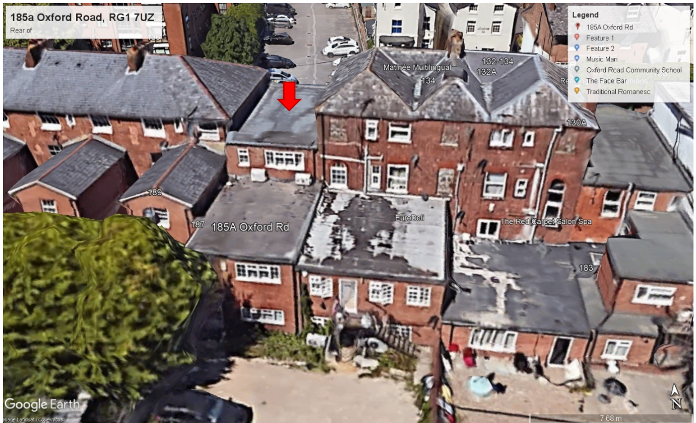
Rear view of the property (Courtesy Google Maps)
