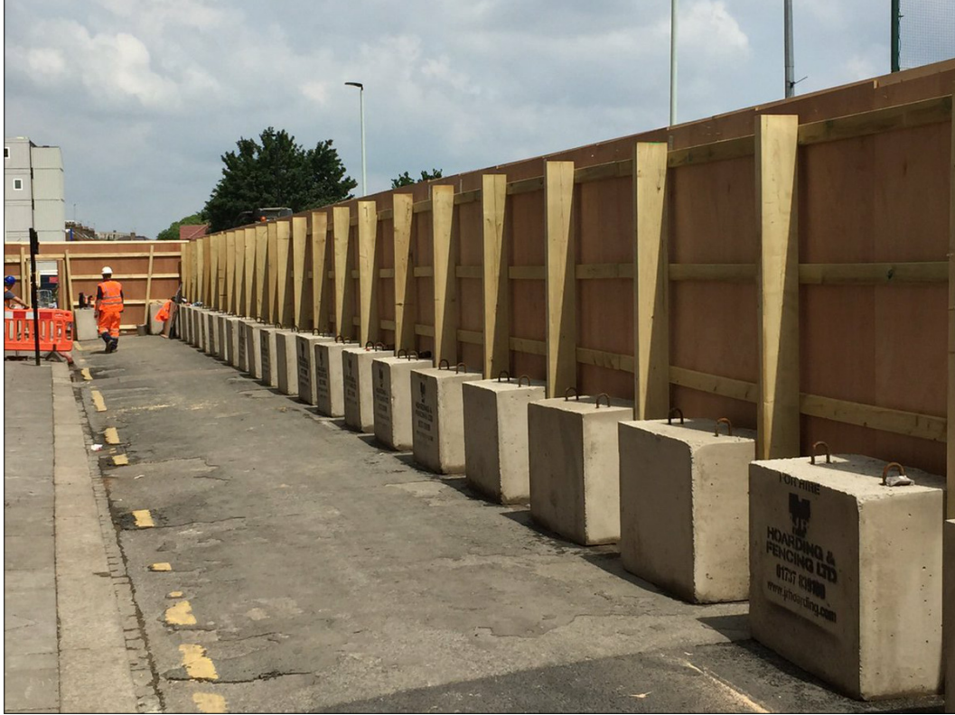
05 TYPICAL IMAGE BALLAST BLOCKS WITH TIMBER UPRIGHTS AND TIMBER HOARDING
