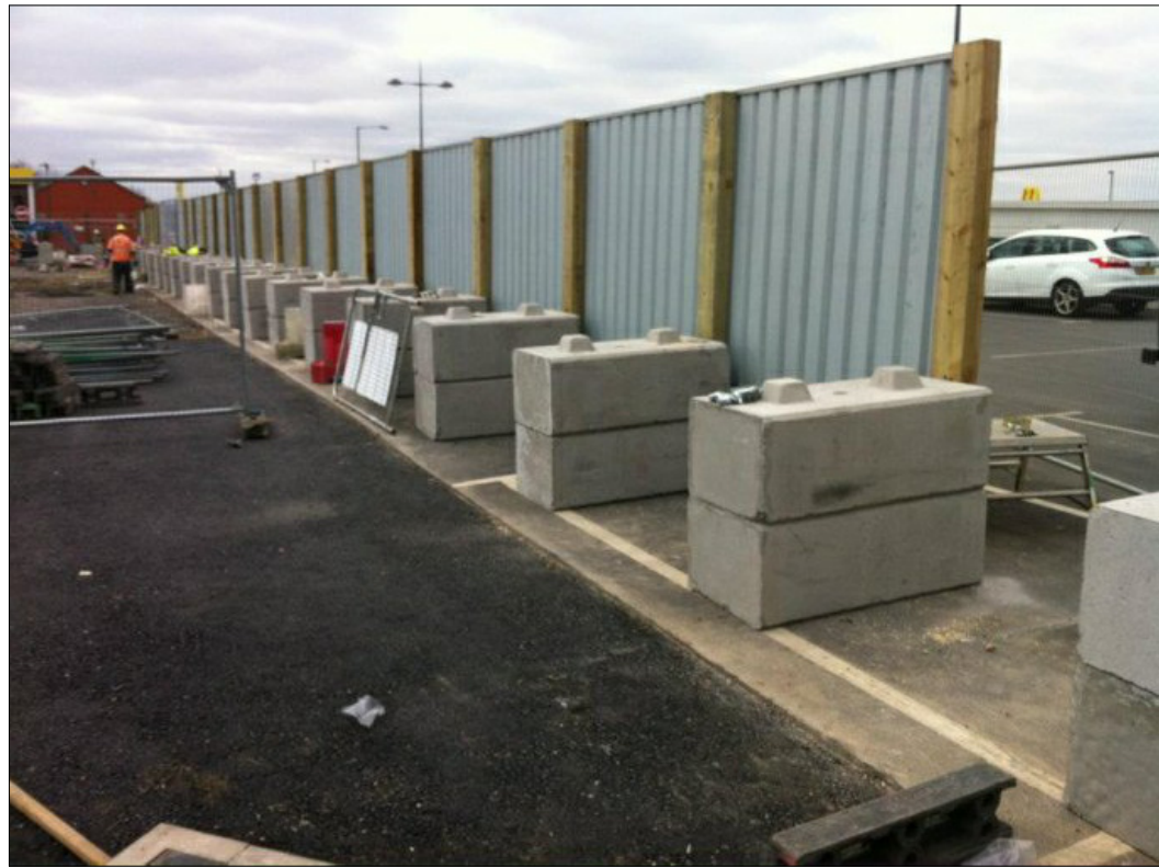
04 TYPICAL IMAGE BALLAST BLOCKS WITH TIMBER UPRIGHTS AND METAL HOARDING
