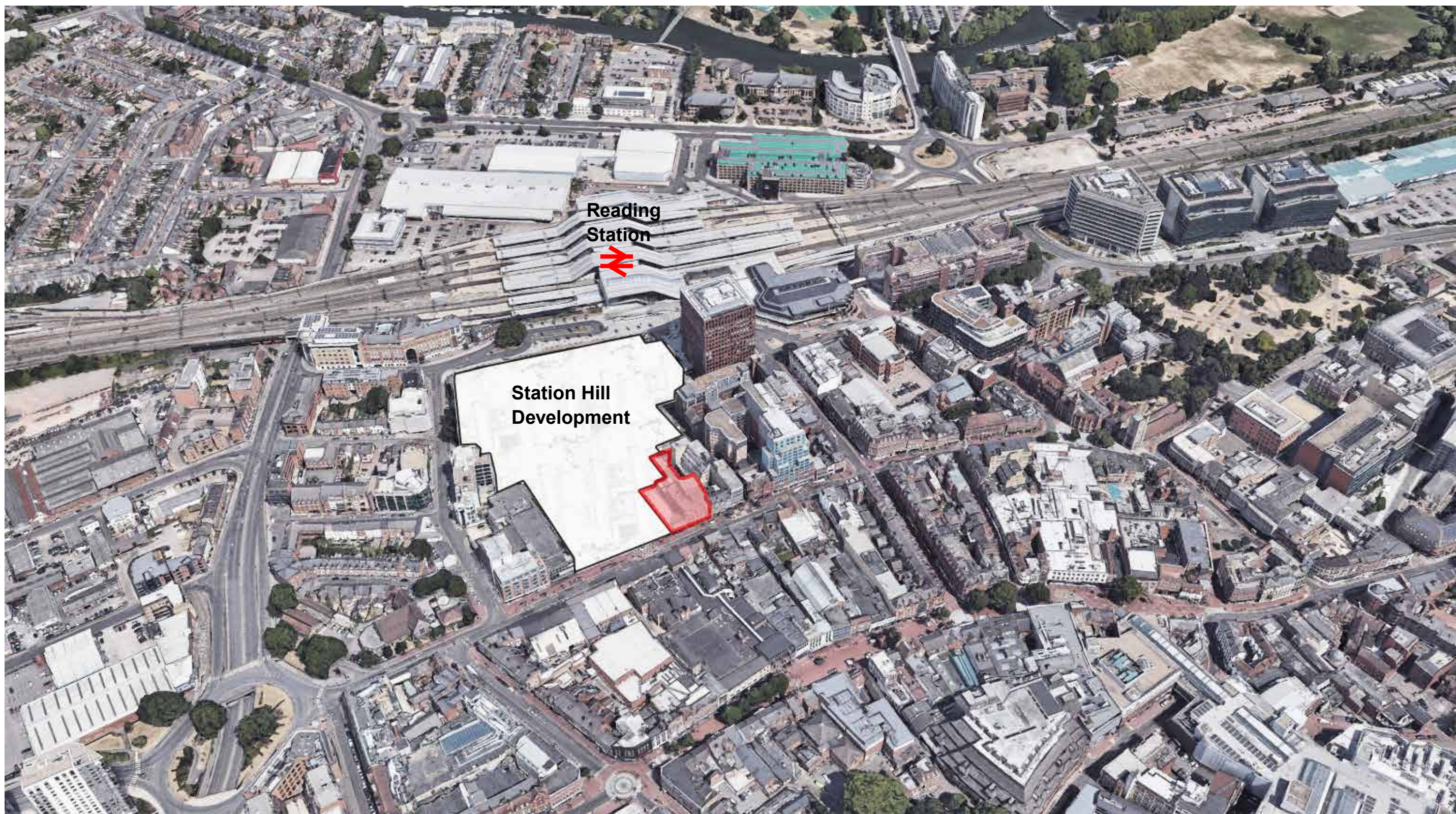
Aerial view highlighting site in red adjacent to the under construction Station Hill Development
