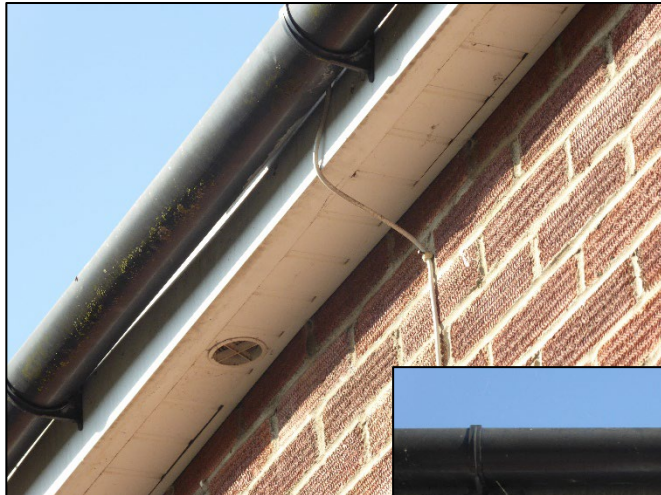
Figure 8. Example sealed soffits and fascias. 1 Briar Close, Caversham. 31.07.24
