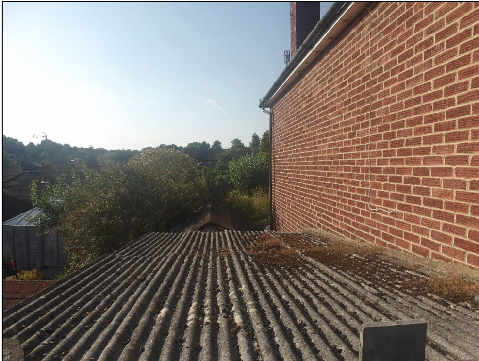
Figure 10. Corrugated sheeting on garage roof. 1 Briar Close, Caversham. 31.07.24
