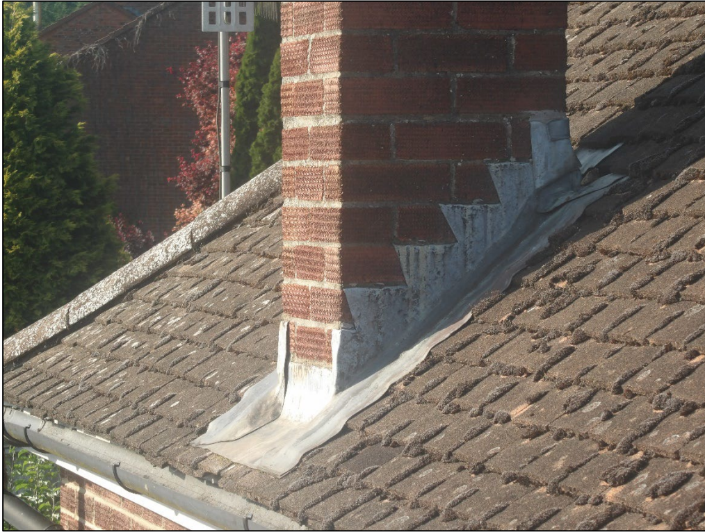
Figure 7. Tightly fitted lead flashing. 1 Briar Close, Caversham. 31.07.24
