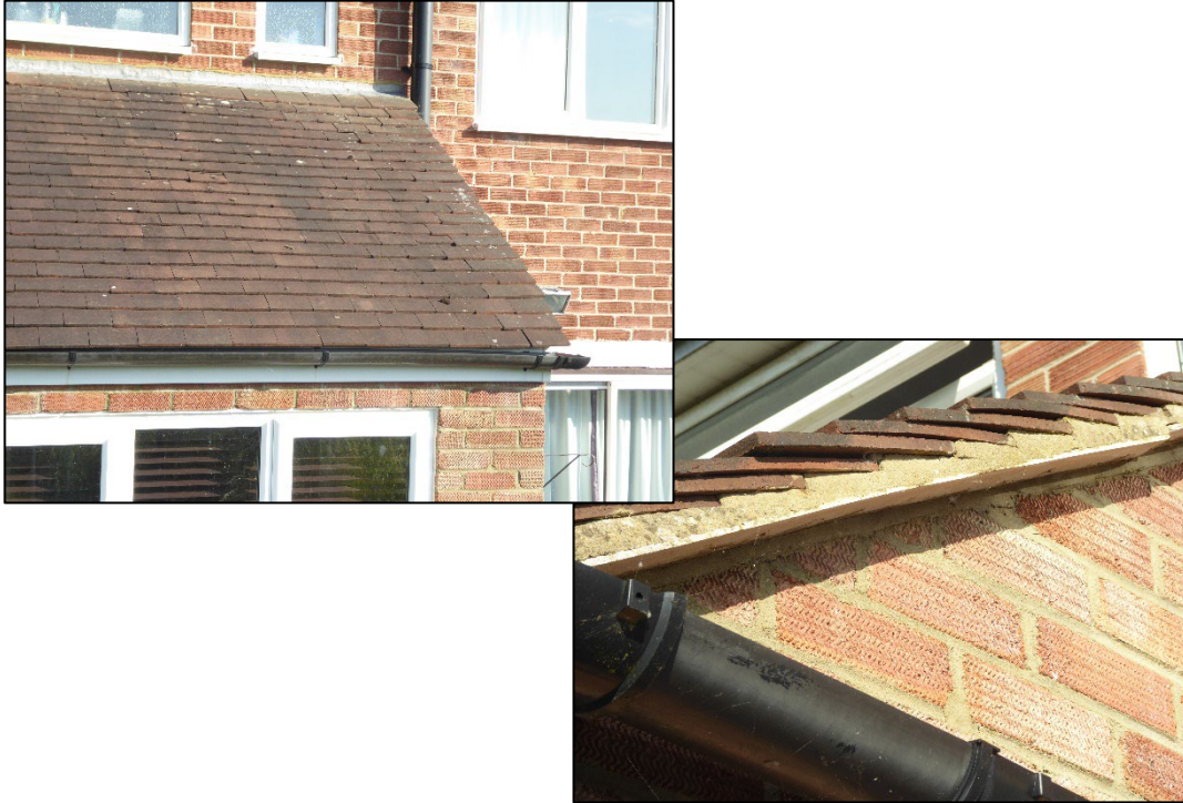
Figure 9. Rear 'lean-to' style roof covering/sealed verges and lead flashing. 1 Briar Close, Caversham. 31.07.24
