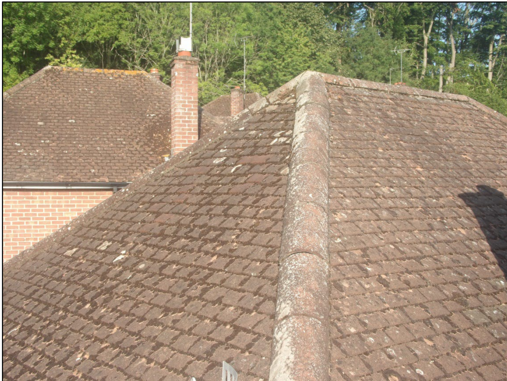
Figure 6. Example ridge and hip tiles. 1 Briar Close, Caversham. 31.07.24
