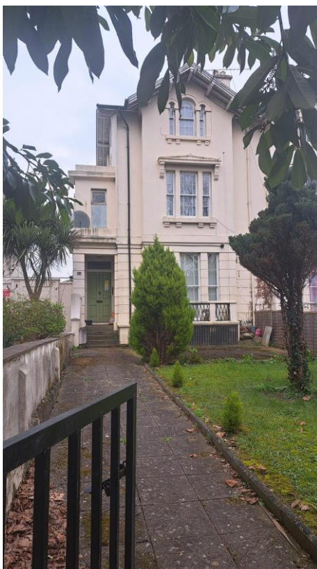
Front elevation of 83 London Road. Image taken by case officer on 7 th March 2024.
