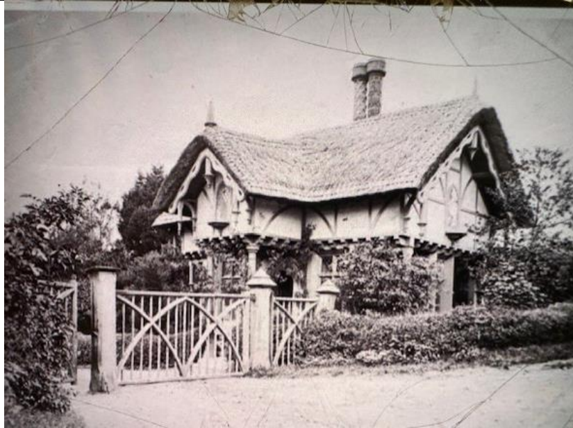
Fig 1: Shows gate across The Warren (Street). No longer there.
