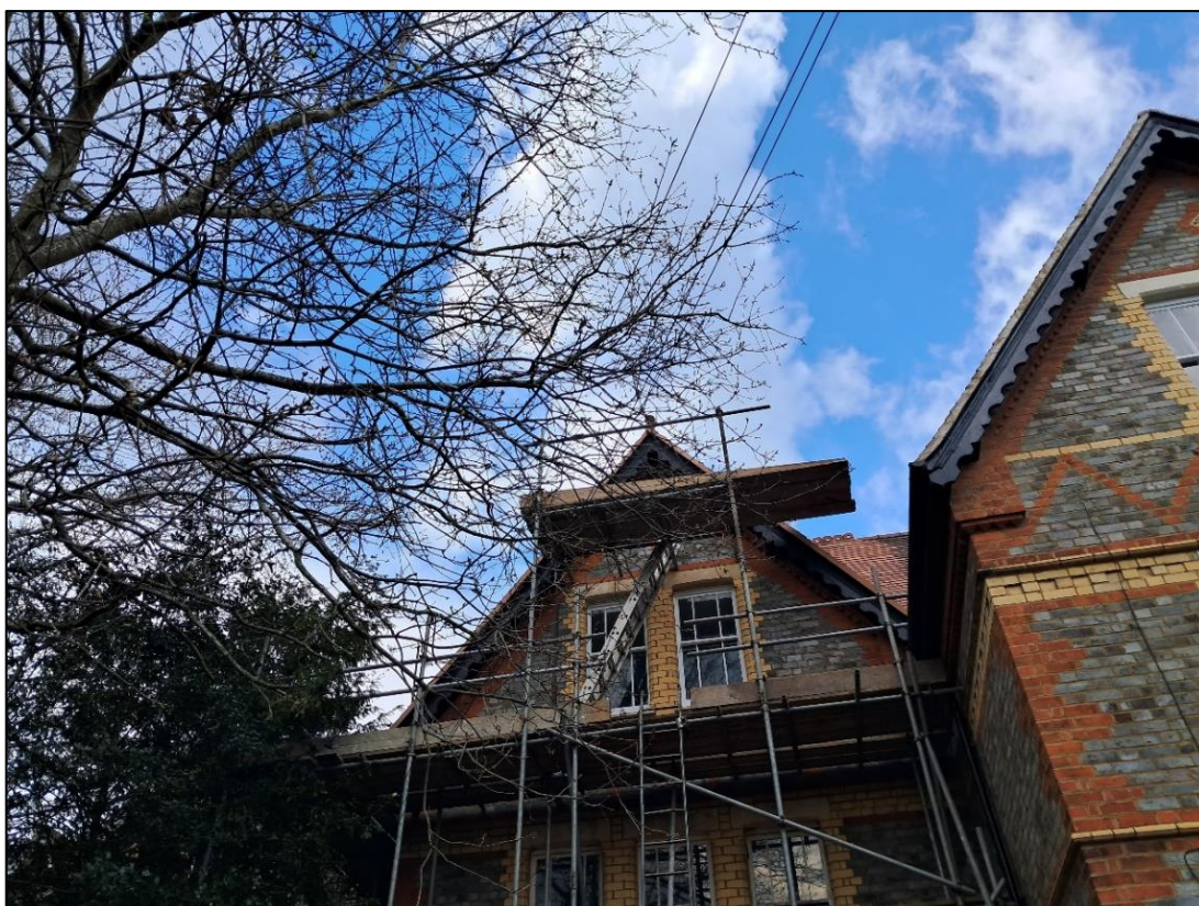
Photo 5 – Canopy of T002 (Oak) prior to permitted works to cut back to clear phone lines in 2023
