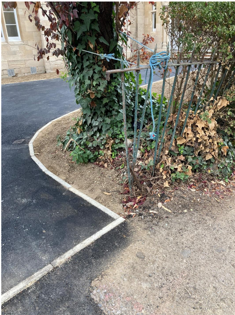
The railings on Craven Road
