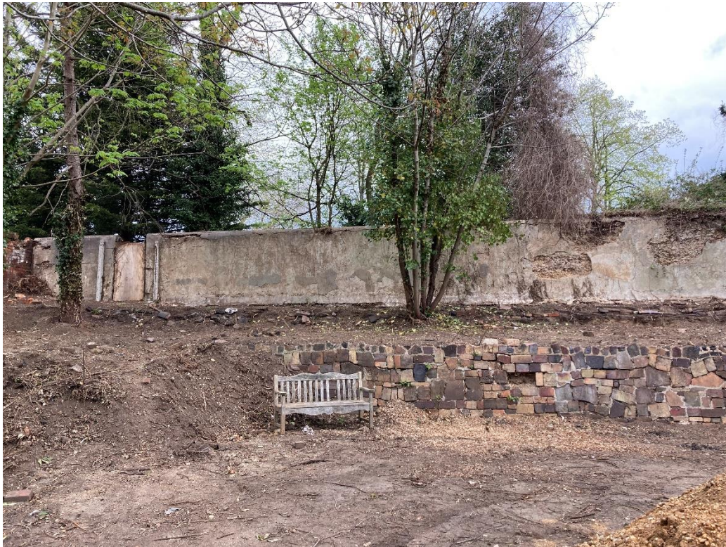
The eastern boundary wall with retaining walls and lower level garden shown after clearance of all scrub
