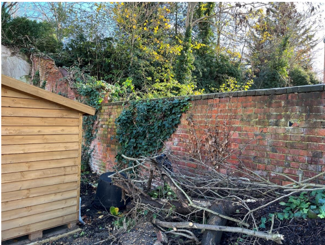
The southern boundary wall
