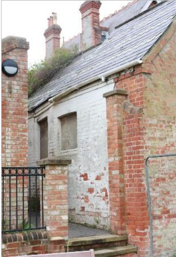
Capped Pilaster at south-east junction
