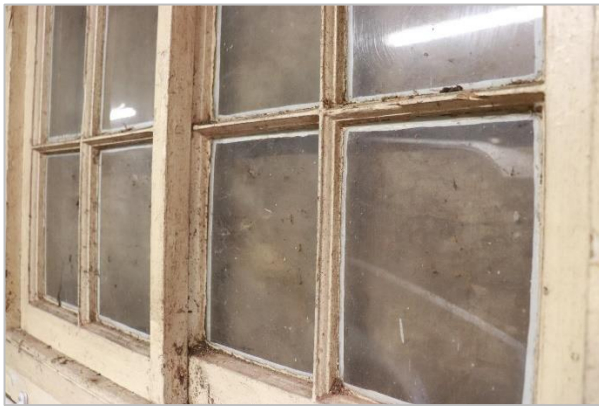
Southern Elevation window detailing
