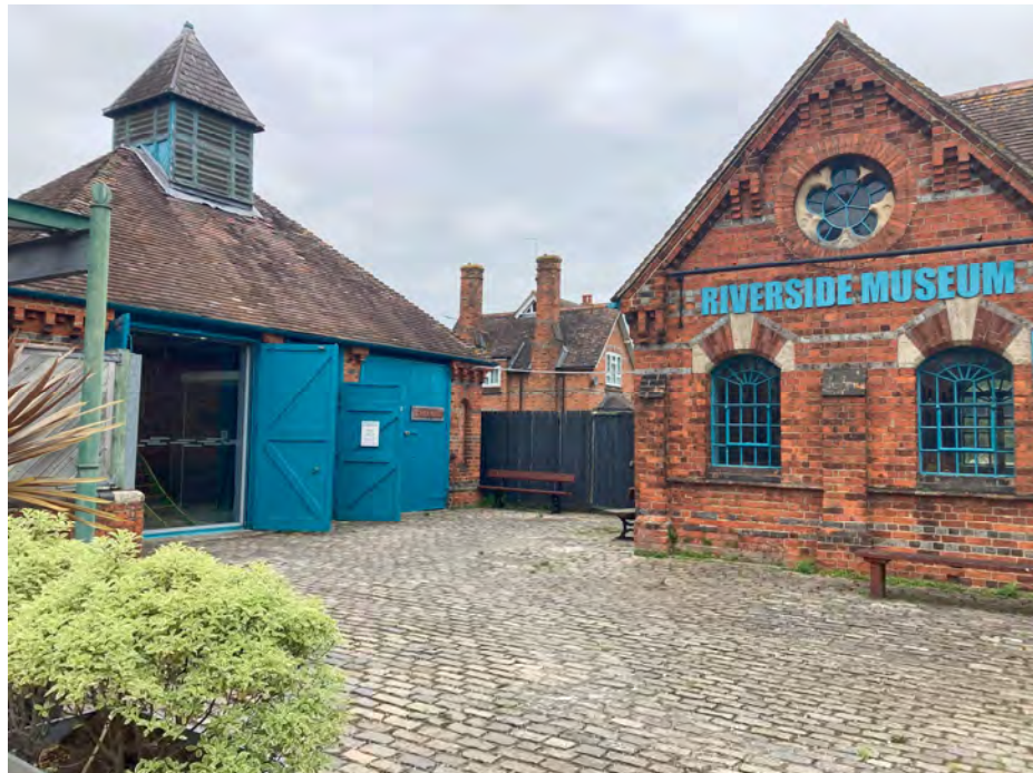
Plate 4 – Adjacent Grade II listed Screens House (left) and pump and turbine house (right).
