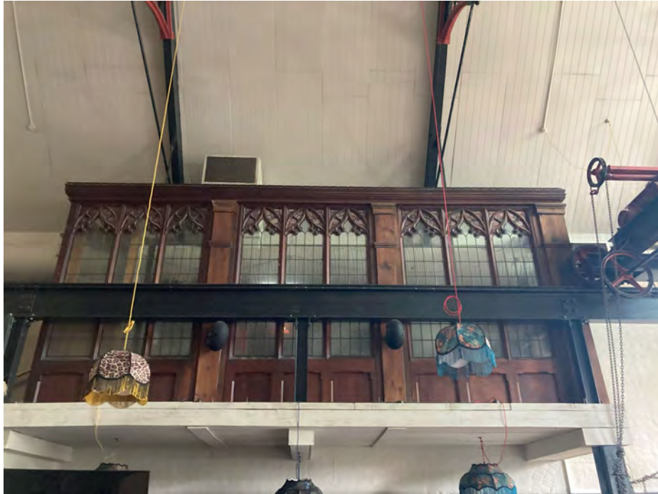
Plate 7 – Mezzanine enclosure to northeast wall of the building.
