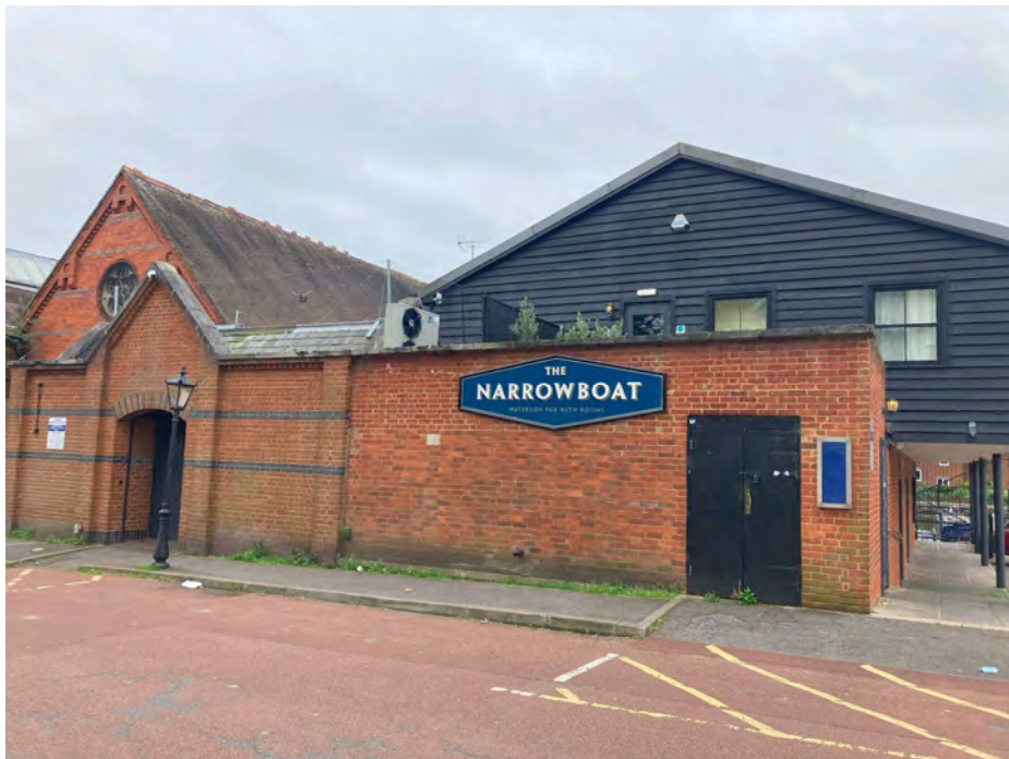
Plate 8 – Rear, northwest elevation onto Gas Works Road; gable end of the former engine house visible to the left of the image.
