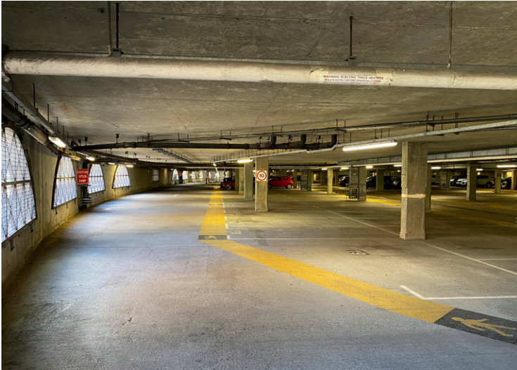
1 - Basement level car park
