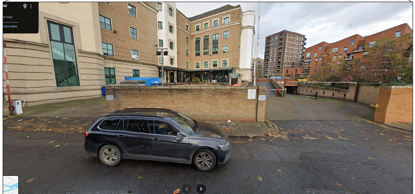
The vehicle entrance to the basement level from Gas Works Road, and external yard where it is proposed the bins are taken on collection days.
