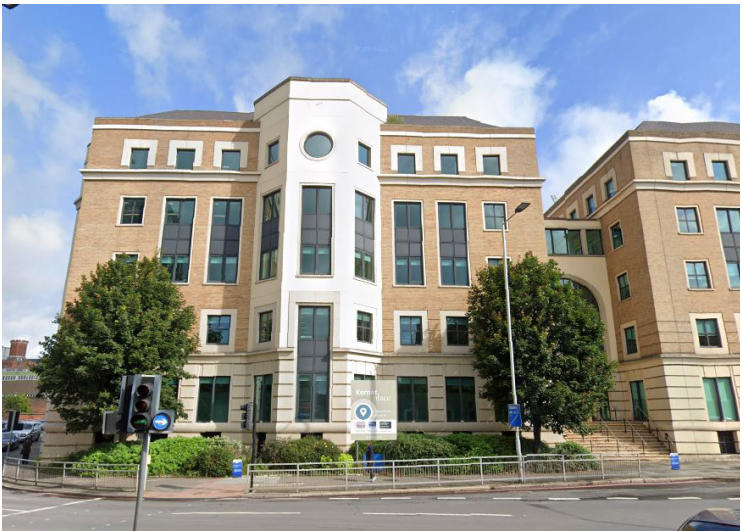
3 - South Elevation viewed from Kings Road
