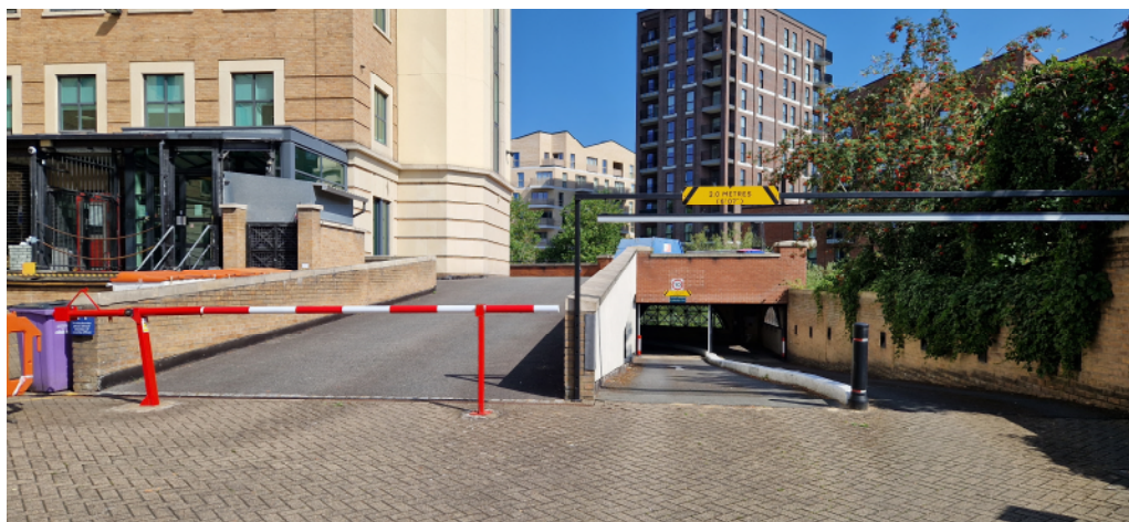
Figure 6: Vehicular Access to courtyard (left) and Car Park (right)
