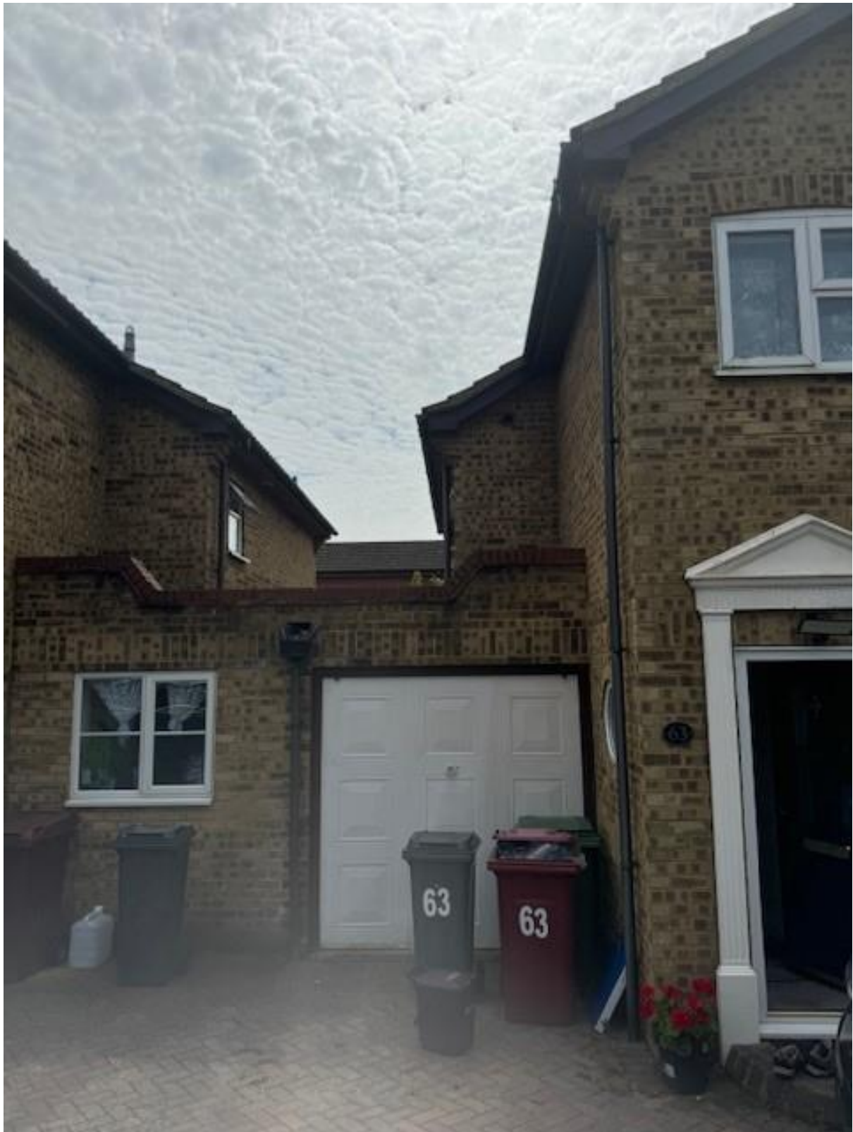
Site Visit Photos as taken on the 31 st of July 2024
