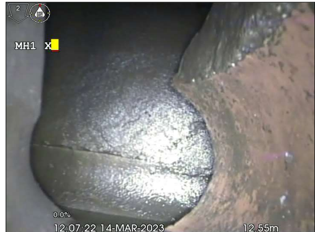
Photo: 2_5a, 00:00:00 12.6m, Finish Survey: MH
