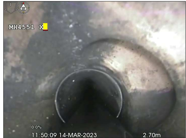
Photo: 60_5a, 00:00:00 2.8m, Junction at 03 o'clock, dia 150 mm
