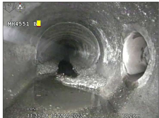
Photo: 83_8a, 00:00:00 19.4m, Junction at 03 o'clock, dia 80 mm
