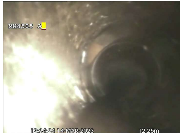
Photo: 6_6a, 00:00:00 12m, Junction at 11 o'clock, dia 150 mm
