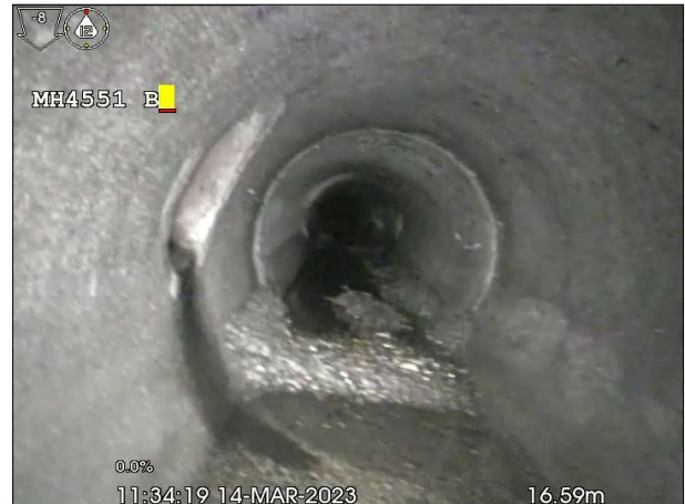
Photo: 81_6a, 00:00:00 16.9m, Junction at 11 o'clock, dia 80 mm
