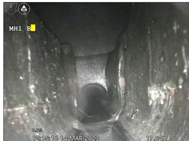
Photo: 4_7a, 00:00:00 17.7m, Finish Survey, Remark: MH1
