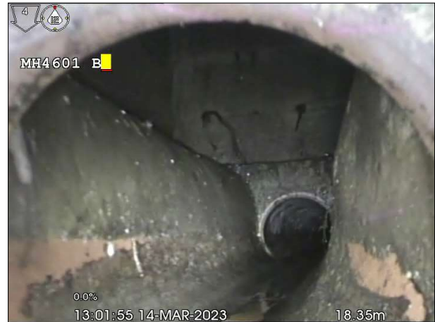
Photo: 100_5a, 00:00:00 18.3m, Finish Survey, Remark: MH
