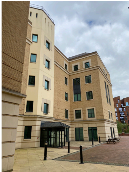
East Elevation, centre and northern wing
