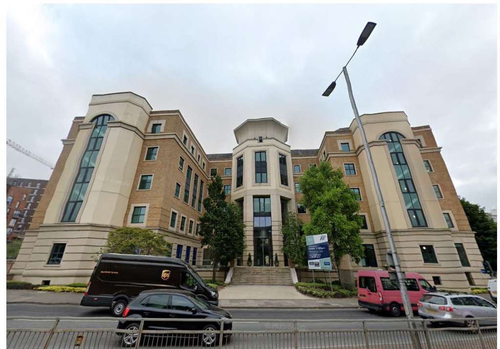
The Front (West) Elevation viewed from Forbury Road
