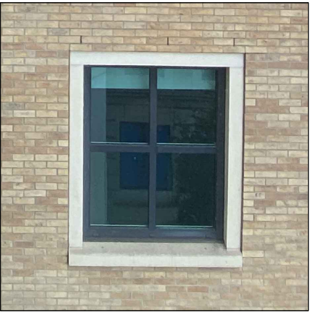
Existing Window Type 02
