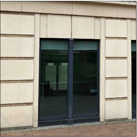
Existing Window Type 03
