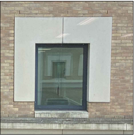
Existing Window Type 01
