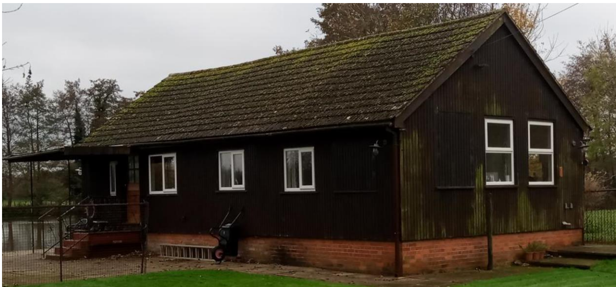
Officer site photograph of the existing building.
