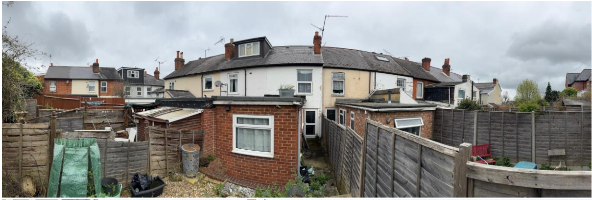
Site visit Photos taken on 11 th of April 2024
