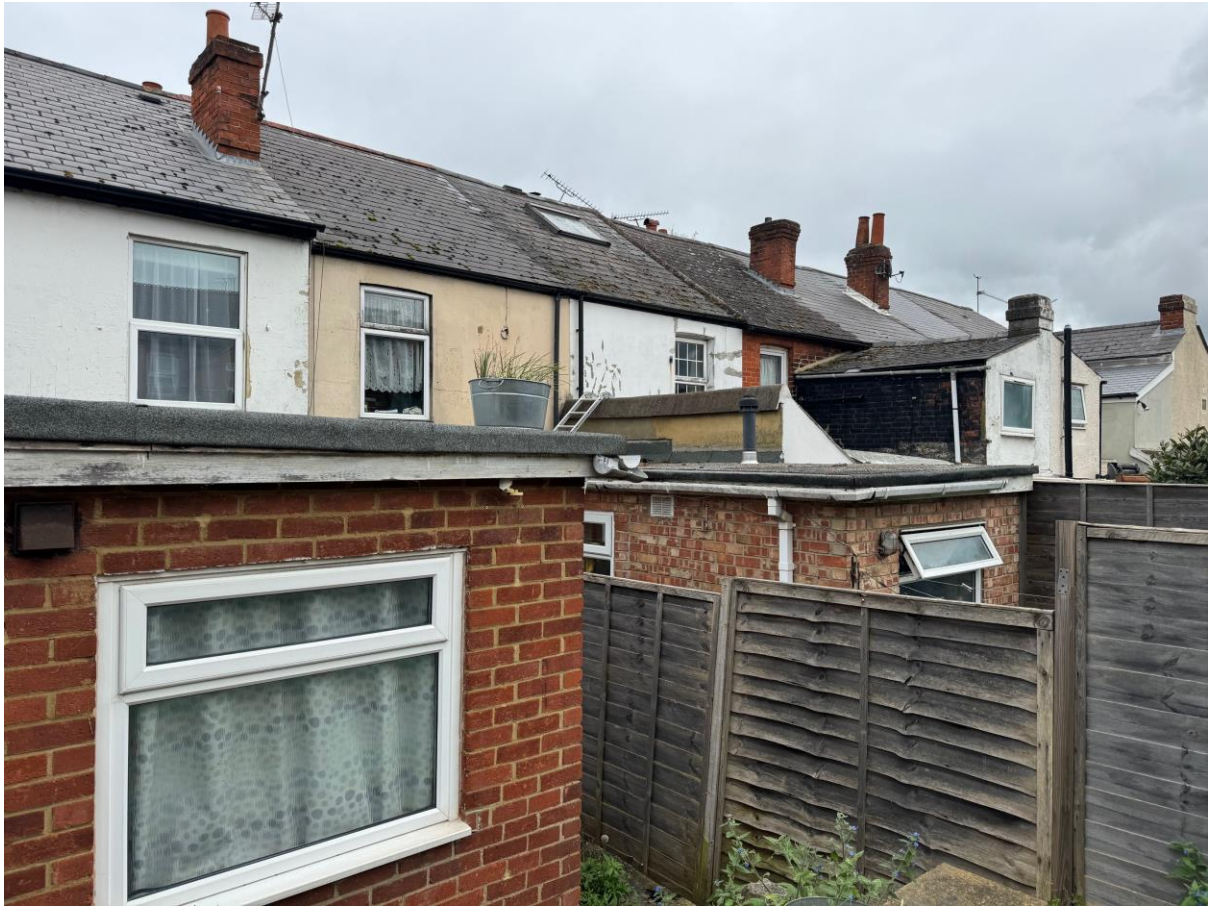
Site visit Photos taken on 11 th of April 2024
