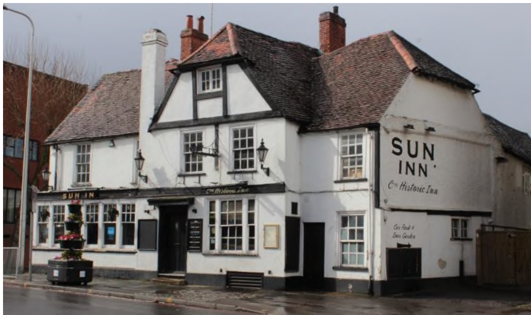
Figure 1 Front and east elevations.
