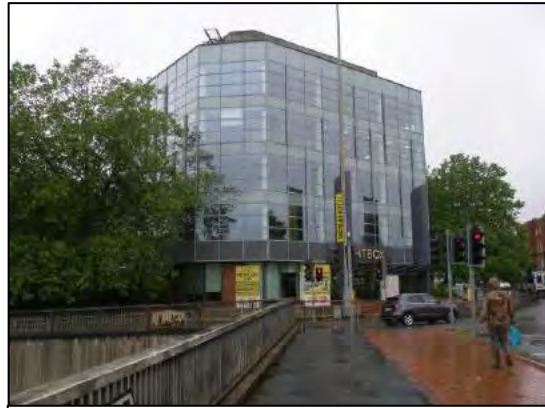
Advantage House view towards west from roundabout
