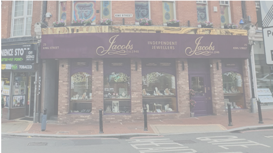
25 KING STREET FRONTAGE JULY 2024
