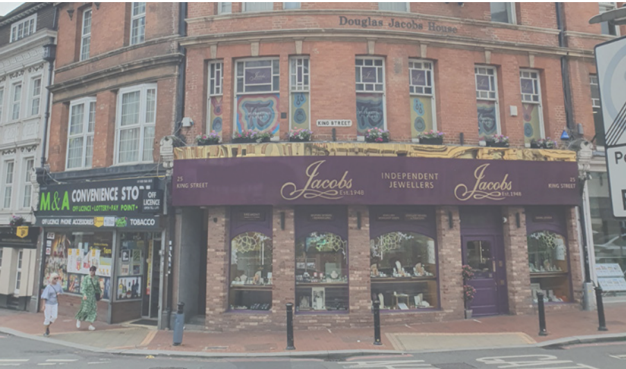
STREET FRONTAGE OF 25 KING STREET AS EXISTING
