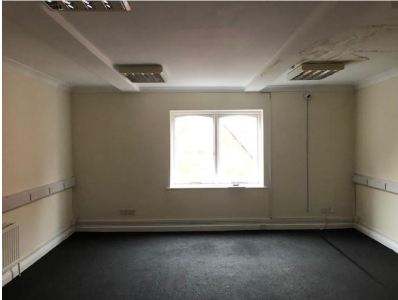
Internal original building
