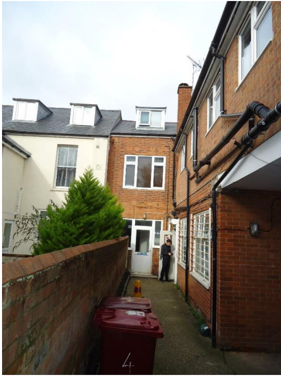
Photo of access to rear of the building
