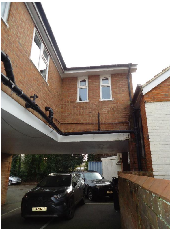
Photo of the car parking in the under-croft at the rear of the building
