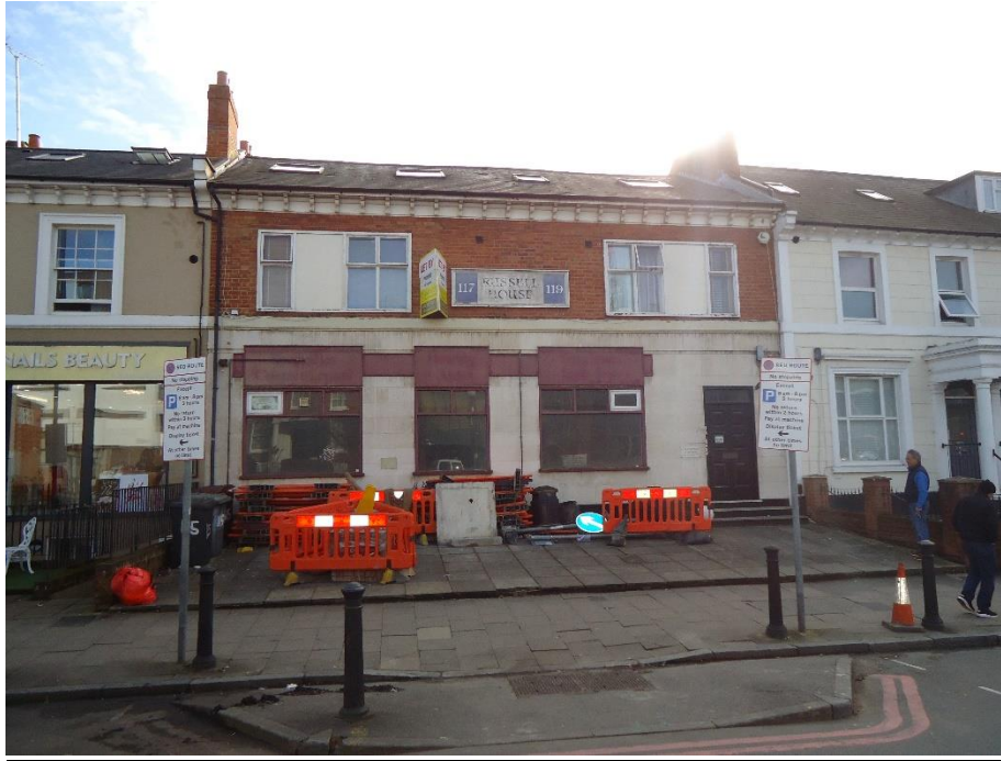
Photo of the existing elevation of the Building
