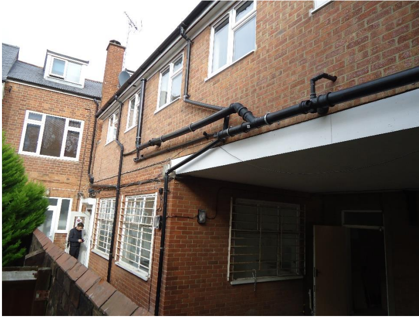
Photo of rear access door to property
