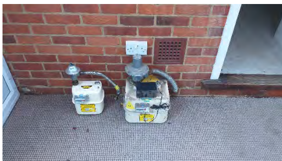
Above, disconnected gas meters inside No.2 Send Road
