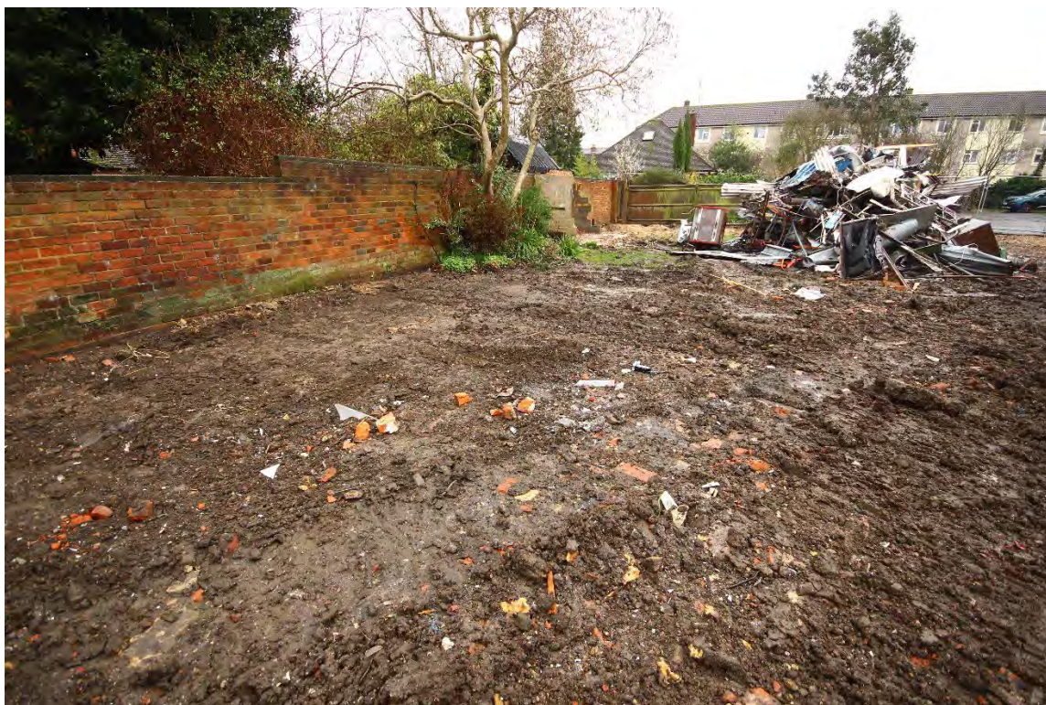
Above, a view of the boundary wall between Ivy Cottage and No.2 Send Road.
