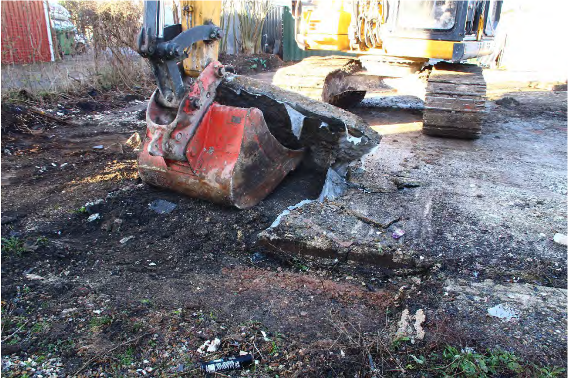
Above, the ground below the Tyre Shop
