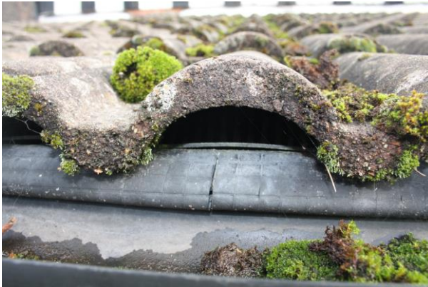
Photo 7: Raised flashing around the intersection of monopitched section
