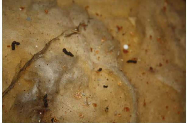
Photo 14: Within the roof void
