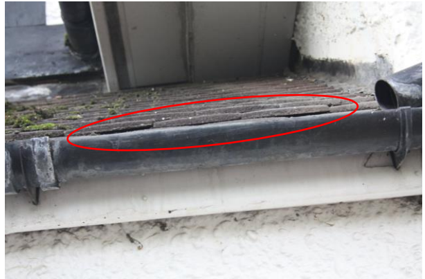
Photo 8: Gaps in soffit box
