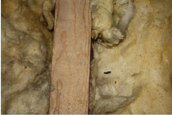
Photo 13: Within the roof void
