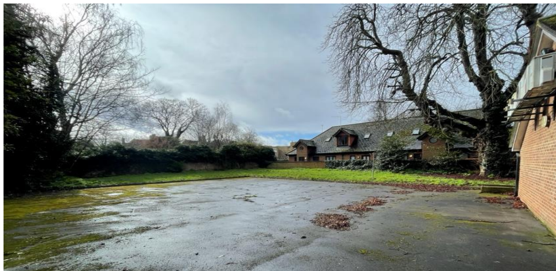
Photo 1: Rear of the site, looking south-west. Showing the developed land; sealed surface.
