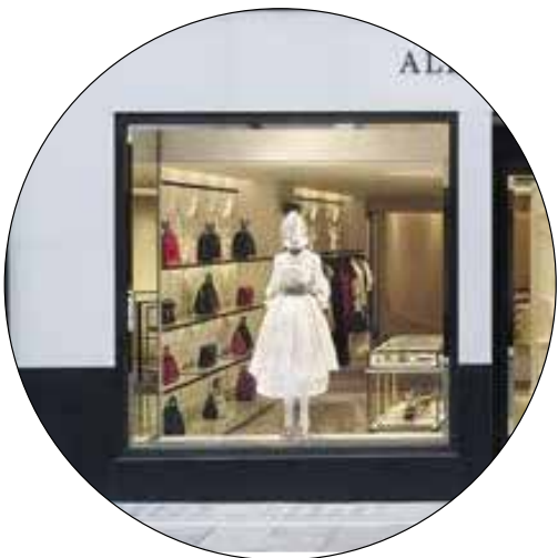
Timber framed shop fronts
