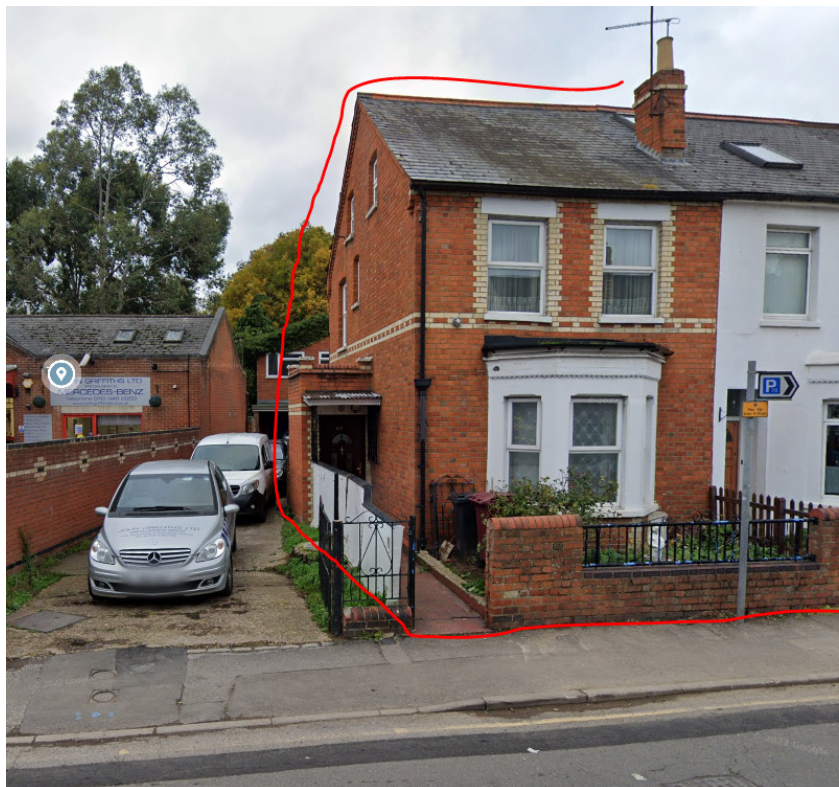
Site visit photograph: 6a Hemdean Road outlined in red
