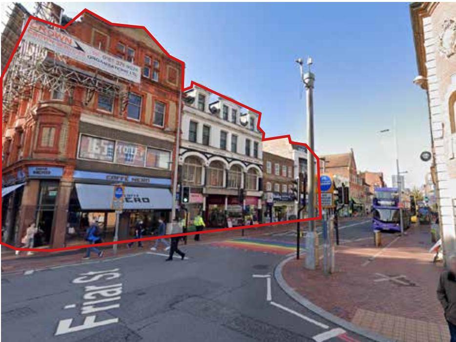
View 03 Taken from Friar Street 145, 146, 147 and 148 (Taken pre-scaffold)
