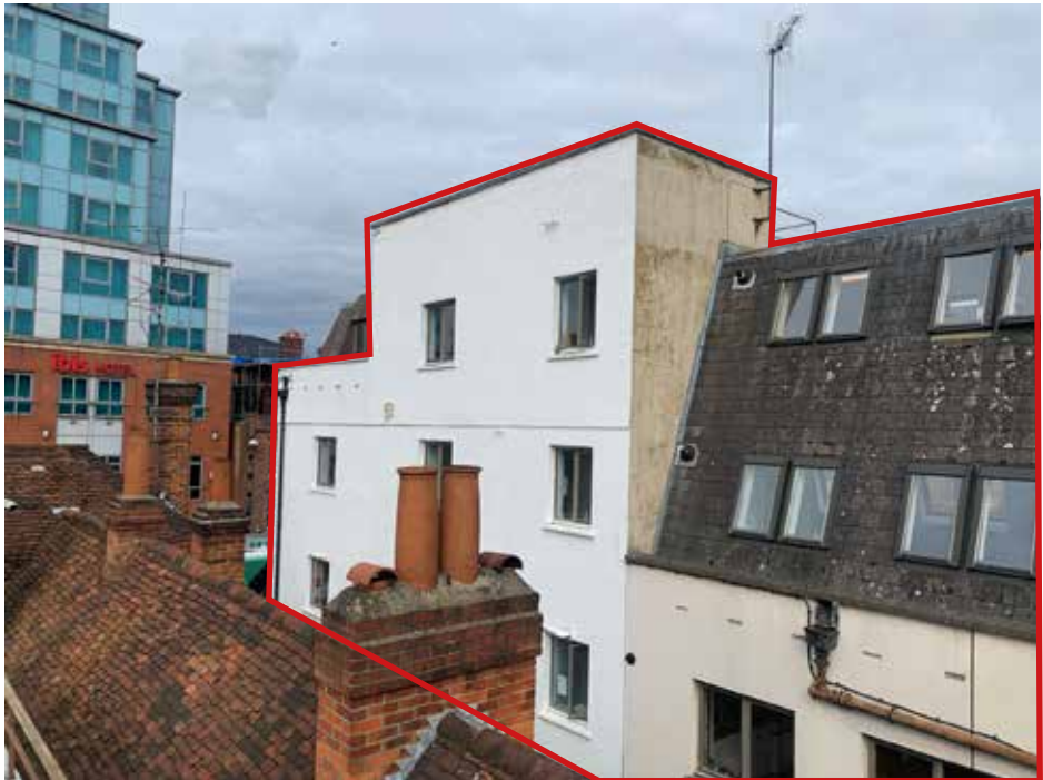
View 02 Taken from roof of neighbouring building capturing upper levels of building 145 Friar Street
