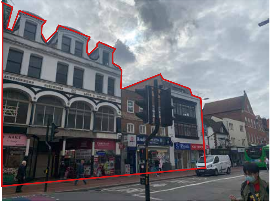
View 03 Taken from Friar Street capturing building 145, 146 and 147.
