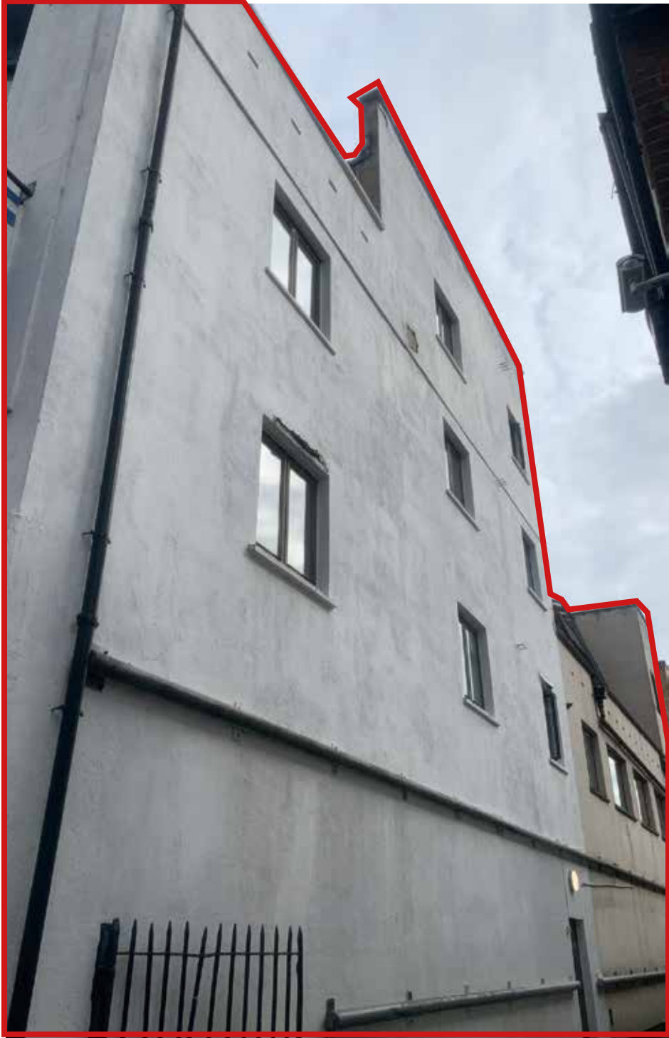
View 03 Taken from Fife Court capturing the side elevation of building 145 Friar Street
