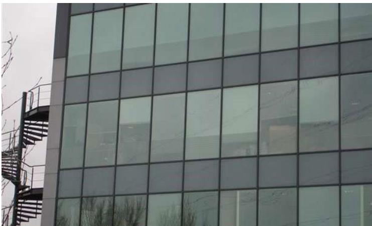
Image 2: Example images of spandrel glazed panels.
