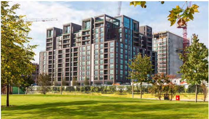
Plimsoll Building, London – David Morley Architects
