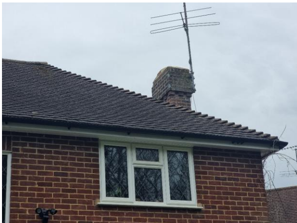
Photograph 3. Detail of the pitched and hipped roof.
