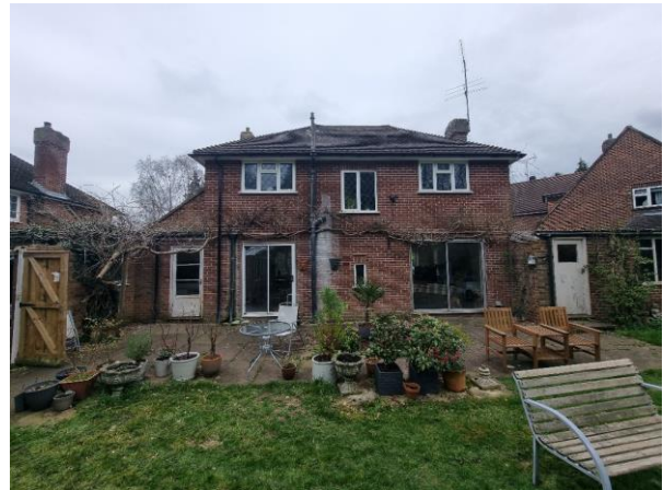
Photograph 2. The eastern elevation of the dwelling.
