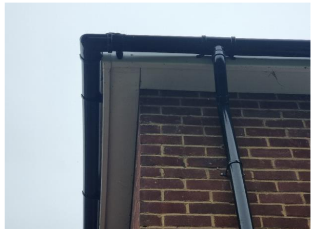
Photograph 4. Detail of the boxed eaves.
