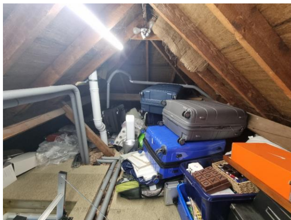
Photograph 10. Detail of the loft space.
