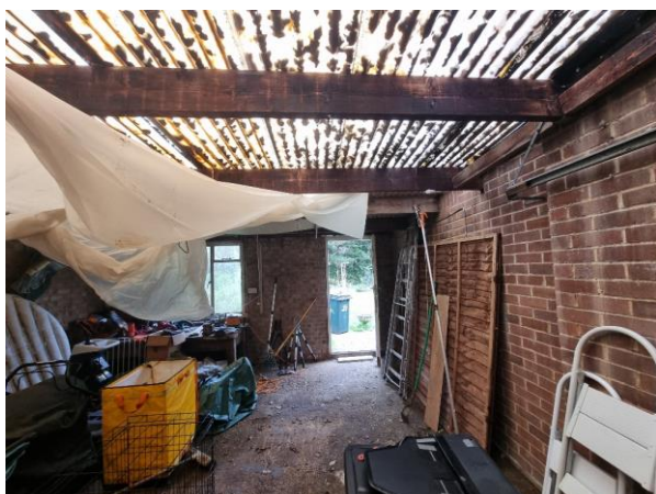
Photograph 11. Internal space of the garage.
