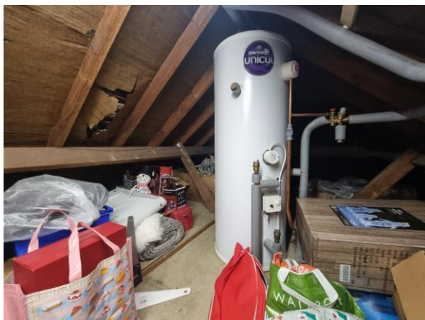
Photograph 9. Detail of the loft space.
