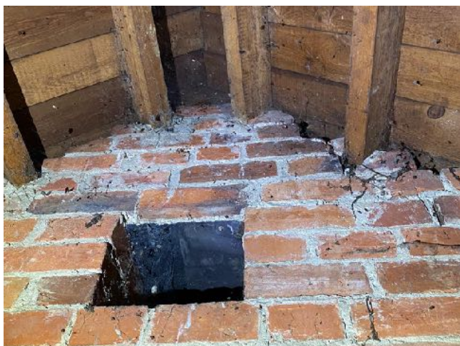
Image 7: Gable end with cobwebbing
