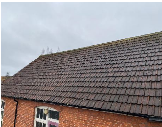
Image 3: Interlocking tiles on northern roof pitch
