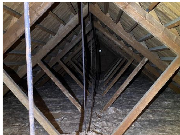
Image 6: Internal loft void looking east
