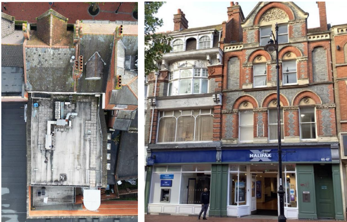
Front Elevation and Arial View drone view.
